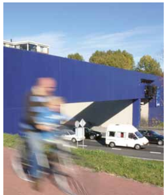
Sijtwende tunnel The Hague, The Netherlands
