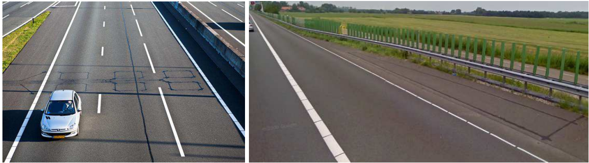
Figure 2.19 Loop pairs in the road surface on a three-lane highway (left) and loop detectors in an emergency bay adjacent to the shoulder lane (right).
