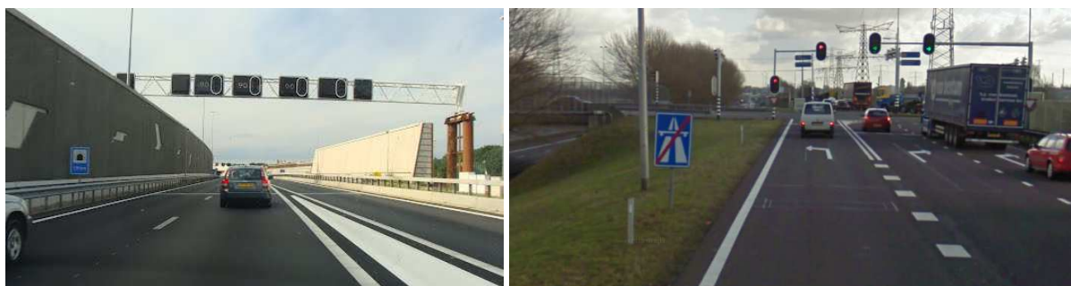
Figure 2.13 Example of traffic lights used at a tunnel (left) and on an intersection at the end of an off ramp (right).
