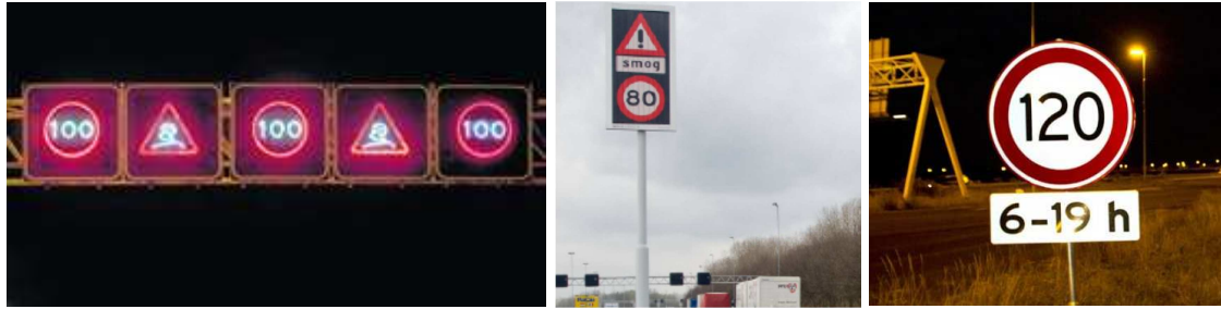
Figure 2.15 Examples of actuators to indicate variable speed limits (left: MSI and additional information signs, center: MUS, right: static road sign with time slot).
