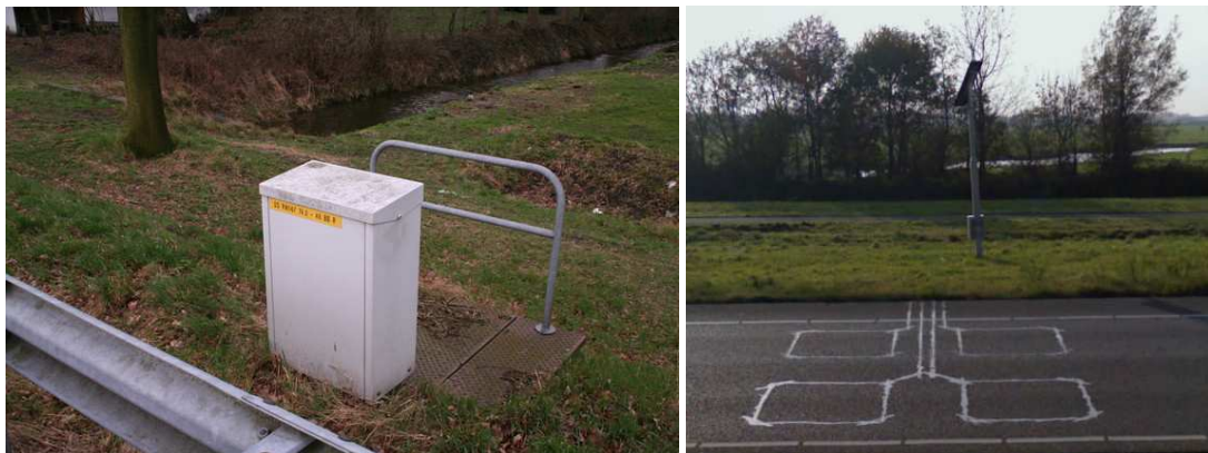
Figure 2.20 MTM detector station (left) and a monitoring detector station (right) placed alongside the road.
