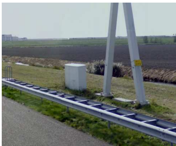
Figure 2.21 MTM outstation near a gantry.
