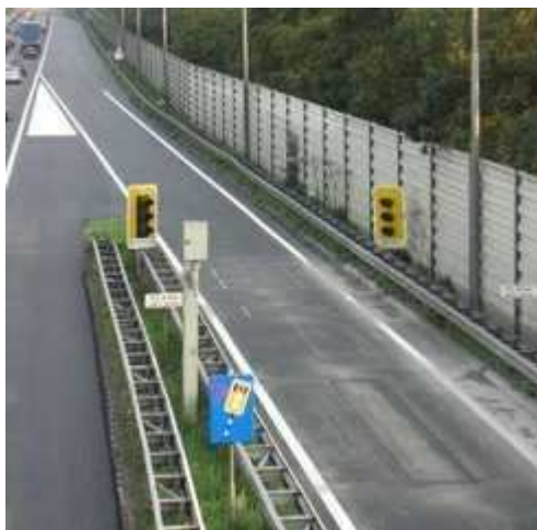
Figure 2.12 Example of ramp metering near an on ramp.
