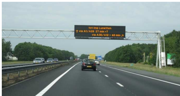
Figure 2.7 Example of a DRIP mounted on a gantry above the road showing travel times on alternative routes.
