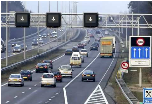
Figure 2.17 Example of shoulder running with a green arrow above the lane and the rotary prism sign indicating the open status of the shoulder lane and the new speed limit.
