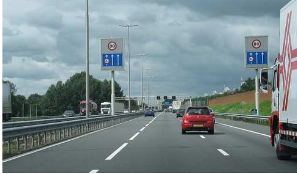
Figure 2.16 Example of a plus lane with rotary prism signs on both sides of the road indicating the use of the narrower lane and the reduced speed limit.
