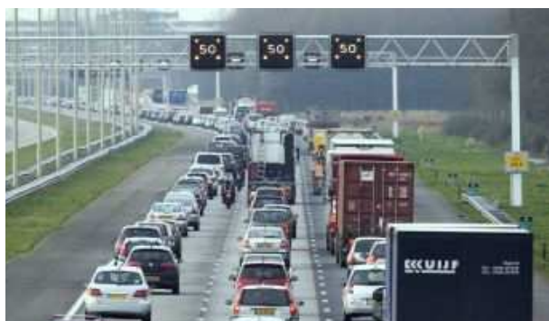
Figure 2.14 Example of MSI above each lane indicating 50 accompanied by flashers to warn for a queue ahead.
