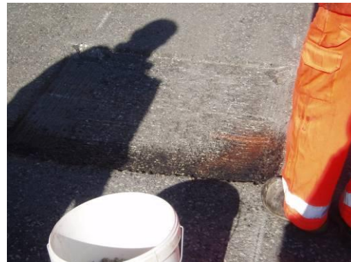
The area is heated with a jet blaster
