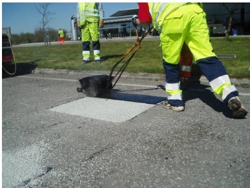
The sealant is applied in a thin layer over the aggregate
