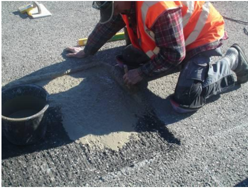
The slurry is distributed with a broom
