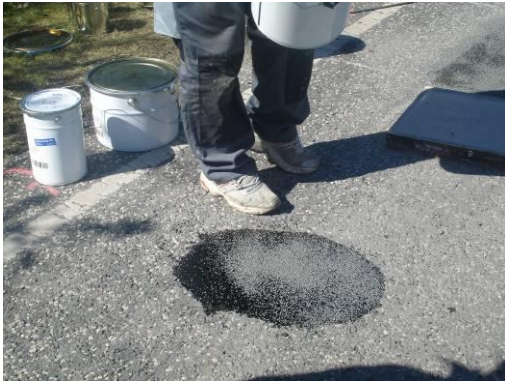
The surface is dusted with aggregate 1-3 mm
