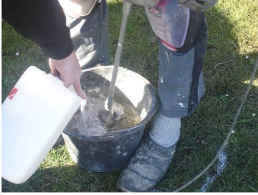
A stapling improver is added until a slurry consistency is achieved
