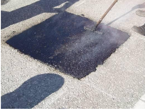
Mastic Asphalt is distributed in the area with a grater
