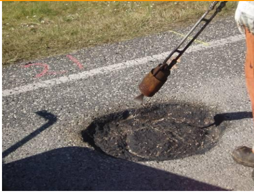
The area is heated with jet blaster
