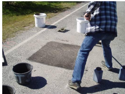
The surface is dusted with sand
