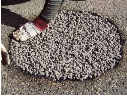
A second layer of steel slag 11/16 mm is added
