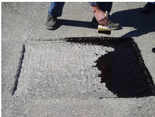
The emulsion is applied with a brush as a primer
