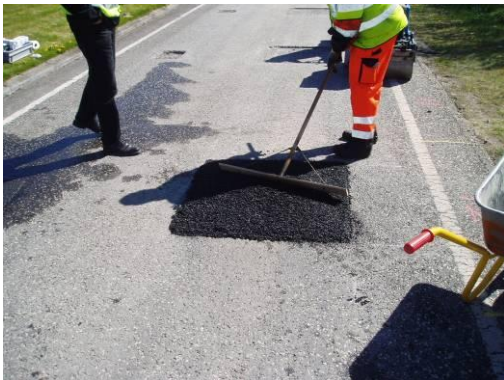
The mix is distributed in the area with a grater
