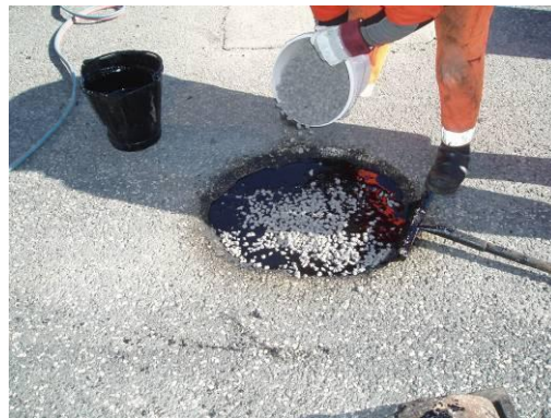
The area is filled with steel slag 11/16 mm
