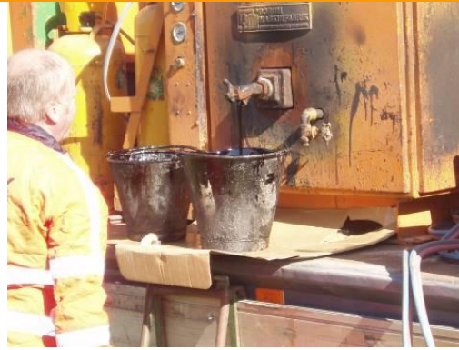
The sealer is tapped from the kettle at 140 °C
