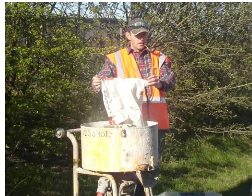
The dry parts are poured into a paddle mixer
