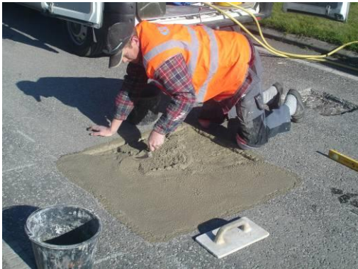
The cement mortar is distributed with a trowel
