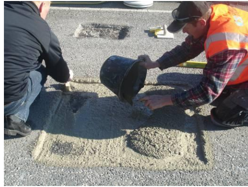
The cement mortar is poured in to the area
