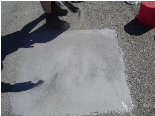
The surface is dusted with aggregate 0,5-1,0 mm
