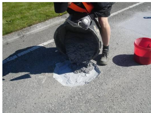
The mortar mixture is poured into the primed area
