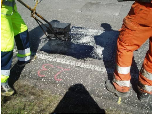
The sealant is laid out side the edge of the area
