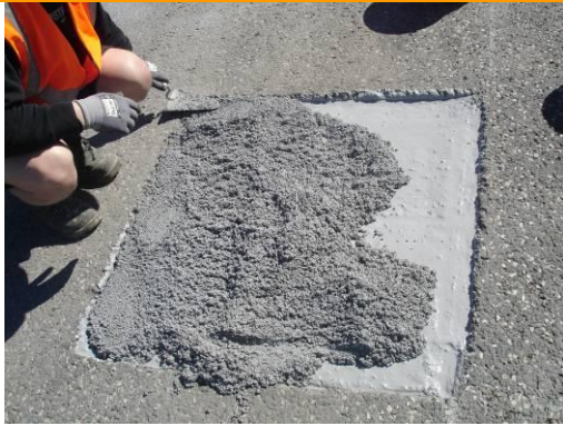
The mortar is distributed with a trowel
