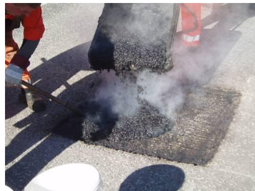
Mastic Asphalt is transferred to the area
