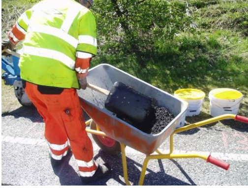
Asphalt and water are mixed with a shovel
