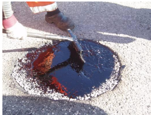
A new layer of sealant is poured over the steel slag
