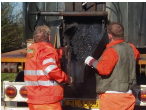
Mastic Asphalt is tapped from the kettle at 224 °C
