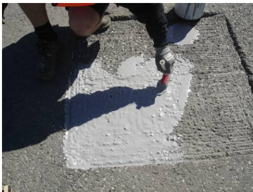
The mixture is distributed as a primer
