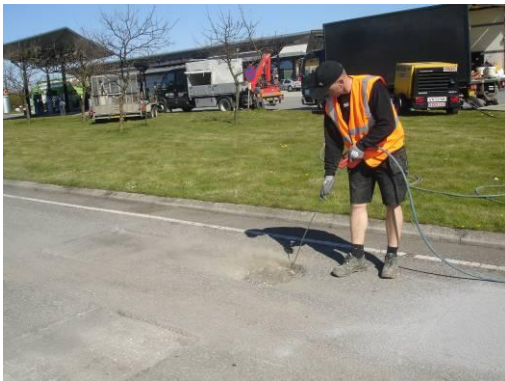
The area is cleaned with compressed air
