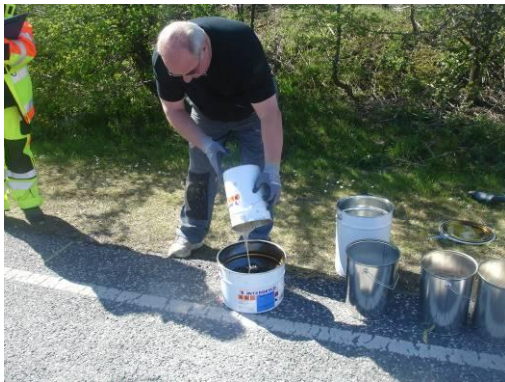
The two components of the synthetic binder are mixed
