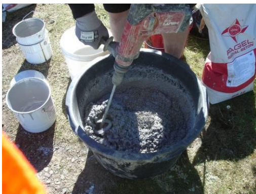
The mortar mixture is stirred mechanically
