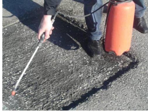
The area is sprayed with tap water
