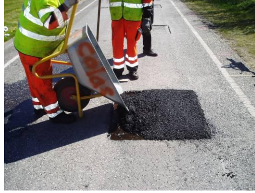
The asphalt/water mix is poured in to the area.
