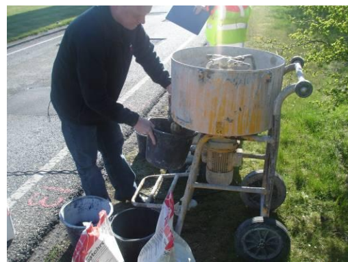
A part of the mix is tapped from the forced action mixer
