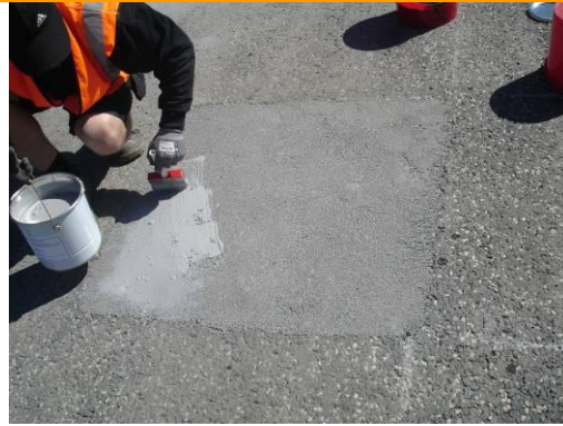
The surface is brushed with a binder mixture
