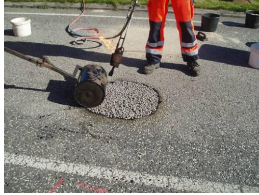
The area is compacted while the surface is heated with a jet blaster
