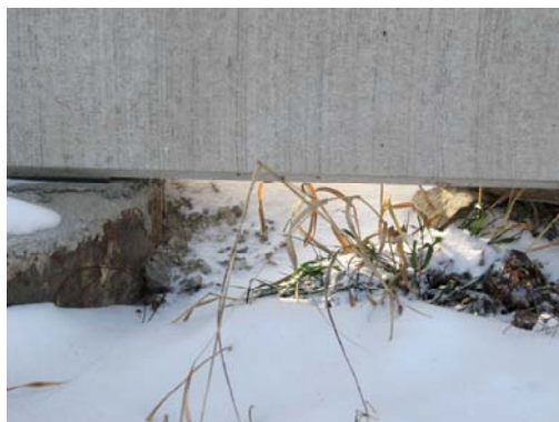
Figure 6: Gap below a noise barrier
