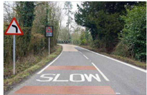
Curve/bend warning sign, SLOW markings, chevron sign, coloured surface and VAS
