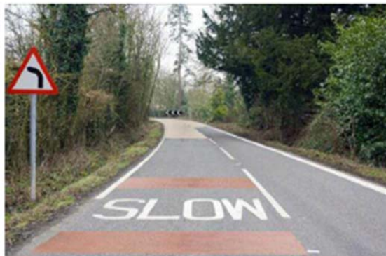
Curve/bend warning sign, SLOW markings, chevron sign and coloured surface
