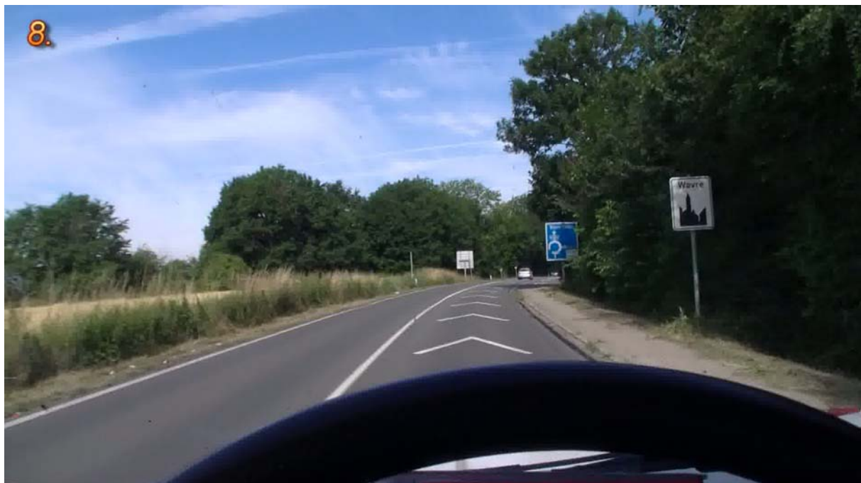
Figure 4: Inappropriate use of chevron markings
