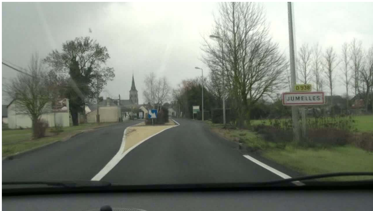
Figure 6: Gate effect combining planting and staggered section that interrupts the visual perspective
