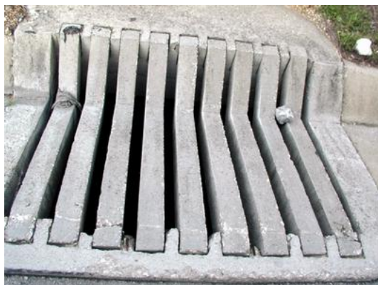
Figure 6.6 – Example of a traversable cross-drainage inlet
