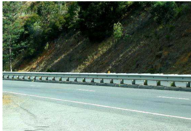
Figure 37: A typical installation of a median W-beam [B.22]
