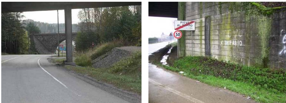
Figure 8: Examples for a hazardous bridge abutment (left) and overpass (right) (Source: [A.2])
