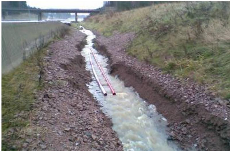
Fig. 20: Excessive runoff, due to heavy rainfall, eroding the top of a drain (Watmove project, 2008).
