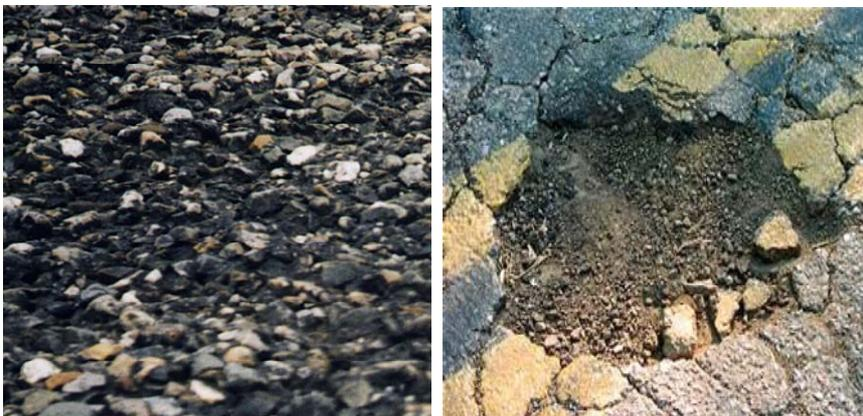
Fig. 4: An example of road subjected to ravelling (left) and to potholing (right) (Watmove project, 2008).
