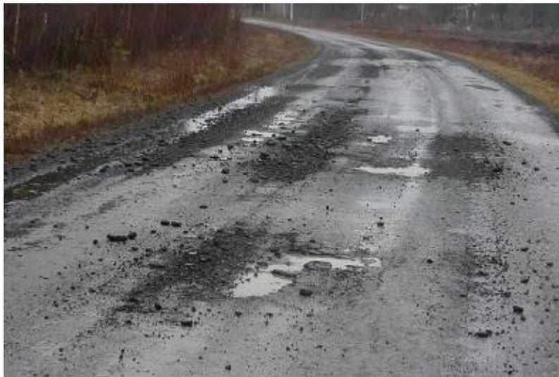
Fig. 1: Road lifted by traffic-induced water pressure during spring-thaw in Northern-Karelia, Finland. Photo courtesy of Martti Leppänen (Watmove project, 2008).
