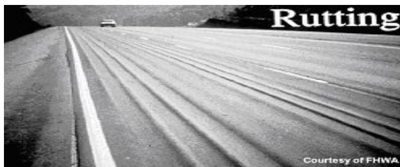
Fig. 5: Rutting of an asphalt road (from FHWA).
