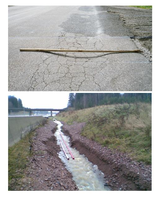
Rutting and cracking of a distressed pavement with poor drainage
