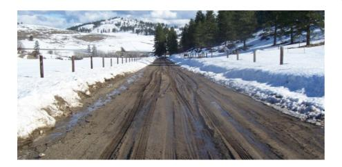
Freezing can pull large volumes of water into an unsealed road which then softens excessively during spring thaw because of inadequate, or impossible, drainage. At the moment the central parts of the Nordic countries experience this during spring. In future they may experience less severe, but longer lasting thaw problems as freezing and thawing occur repeatedly in a warmer winter
