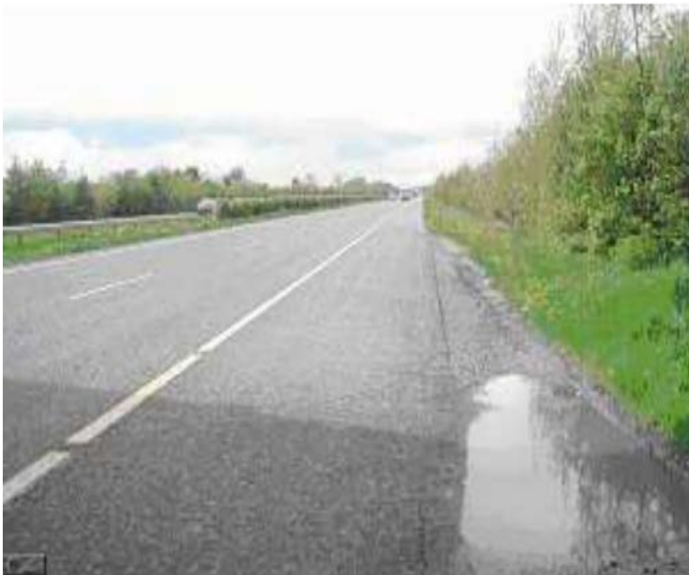
Figure 27. Filter drain ponding on the Maynooth M4 site.
