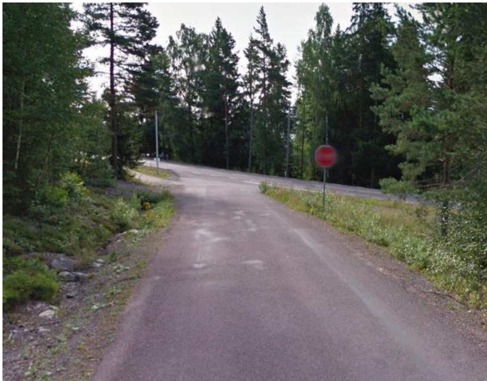
Figure 31: Poor visibility of cycle facility from side road
