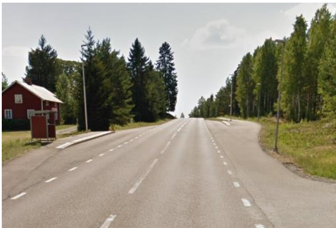
Figure 29: No clear definition of cycle facility (right hand side of image)
