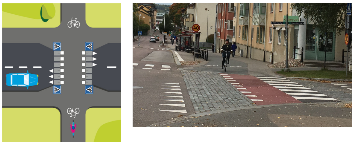
Figure 28: An unsignalized bicycle-priority crossing in Sweden, in theory (left) and an example from real-life (right).
