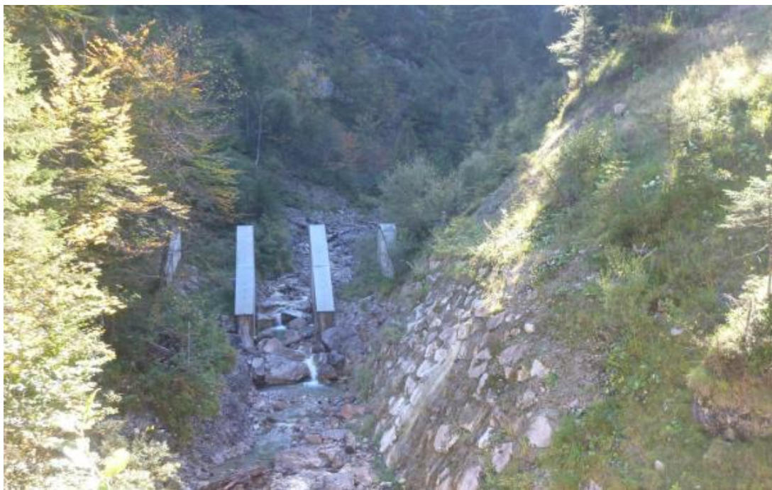
Figure 2.9: Mudflow breaker, to reduce the energy of a flood with heavy stindes or high speed
