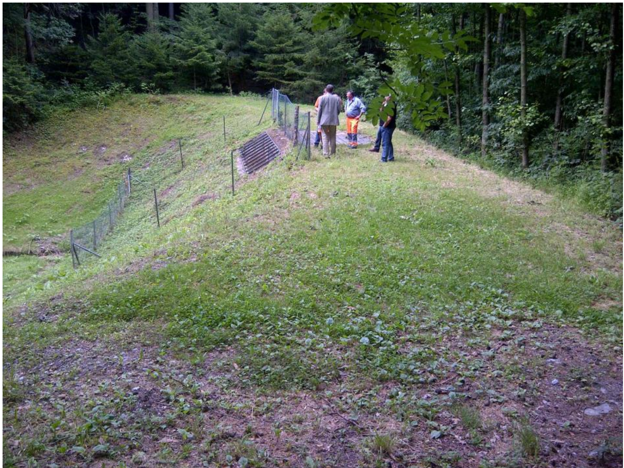
Figure 2.3: Dam of a flood retention basin
