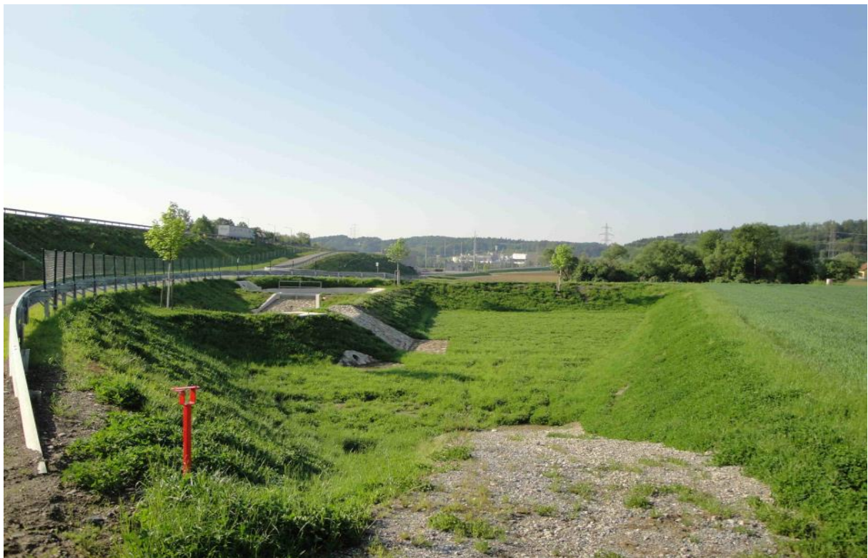
Figure 2.1: Water treatment plant (sedimentation basin, infiltration basin)
