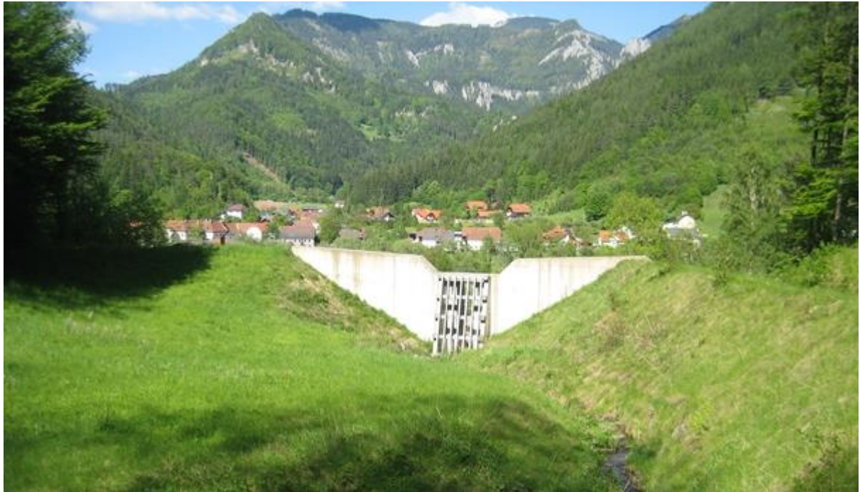
Figure 2.5: Bedload barrage, against mudflows
