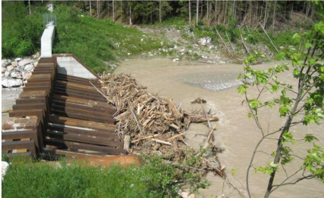
Figure 2.8: Wild wood rake, to protect pipes and small bridges
