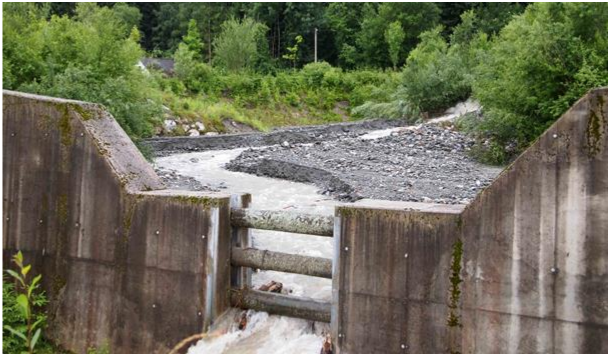
Figure 2.6: Bedload barrage, against mudflows
