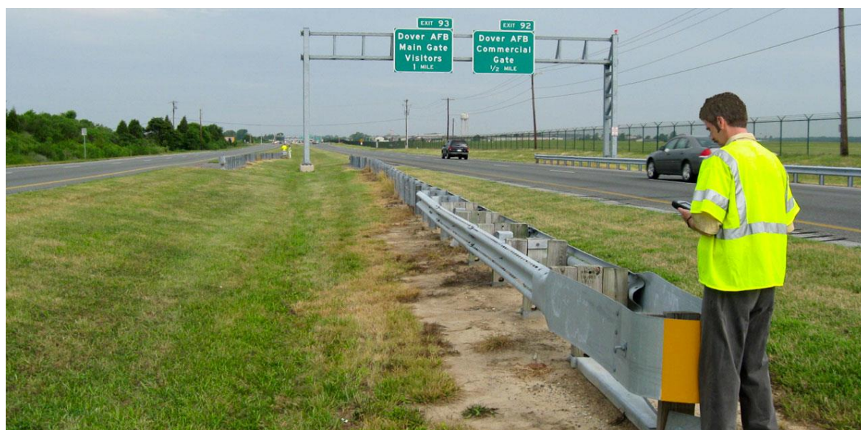
Figure 10: Manual inspection of VRS
