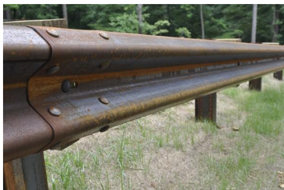
Figure 14: Rust on the front side of VRS
