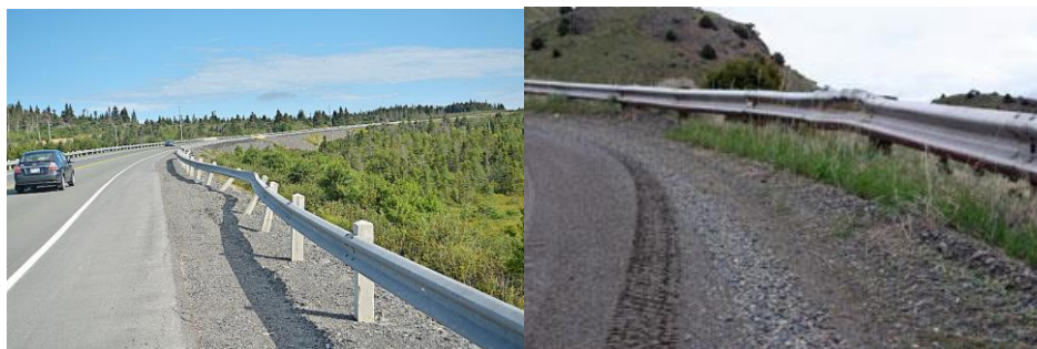
Figure 13: Examples for damaged VRS (visible from Video)
