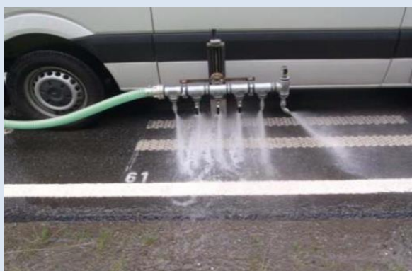
Figure 42: Spraying system with nozzles
