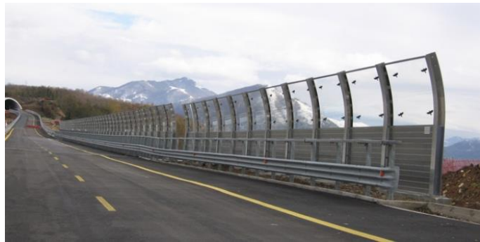
Figure 40: Noise barrier and vehicle restraint system
