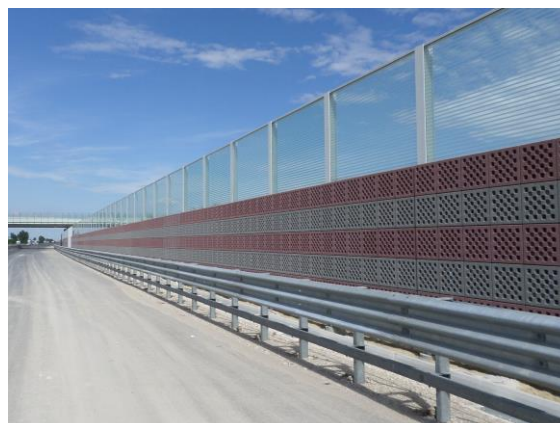
Figure 9: Noise barrier protected with VRS
