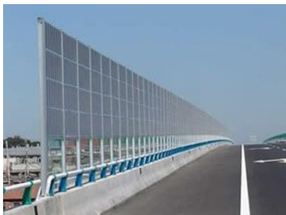
Figure 8: Example for noise barrier, where inspection may be dangerous
