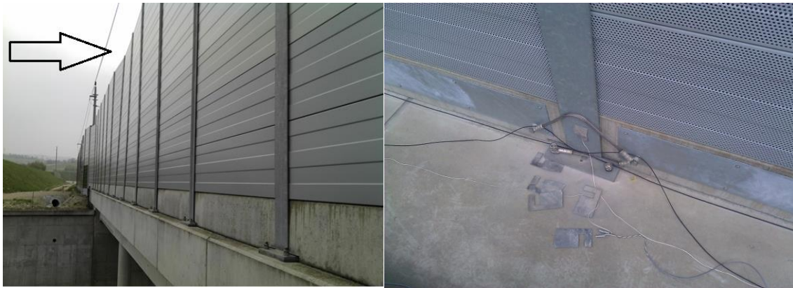
Figure 38: Visual inspection detect obvious defect (left) and dynamic measurement (right)
