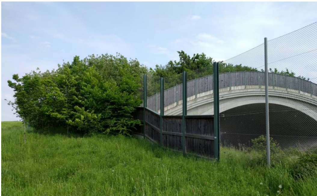
Figure 4 - Fences and screens must be very tightly connected as even small gaps may divert the bats away from the overpass and onto the road (Photo by SWILD & NACHTaktiv).
