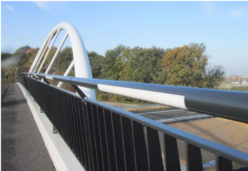
Figure 11 - Lighting on this bicycle bridge in the Netherlands has been installed in the railing to reduce the light spillages into the surroundings and maintain a dark zone along the bridge to encourage the bats to use it as a safe overpass (Photo by V. Loehr).
