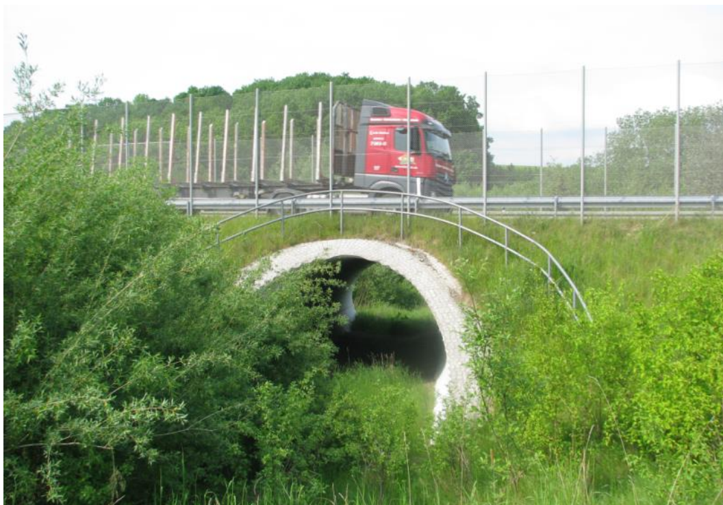
Figure 8 - Hedgerows have been planted to guide the bats into the tunnel under the state road S170n in Germany. Tall fences on the road above the underpass enhance the effectiveness of the passage for low-flying species and may function as a hop-over for species with medium and high flying heights (Photo by SWILD & NACHTaktiv).
