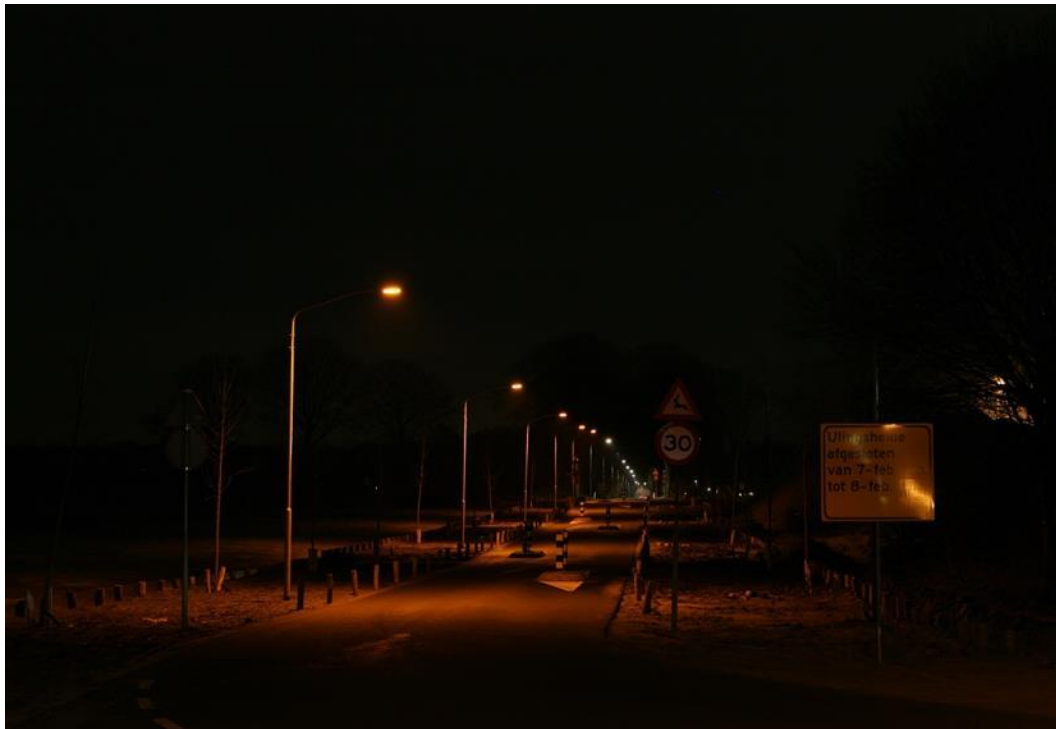
Figure 10 - The amber coloured street lighting may minimise the light disturbance of bats. Furthermore, the lamps on this path in the Netherlands are only switched on when there is a bicycle or a pedestrian on the road (Photo by V. Loehr).
