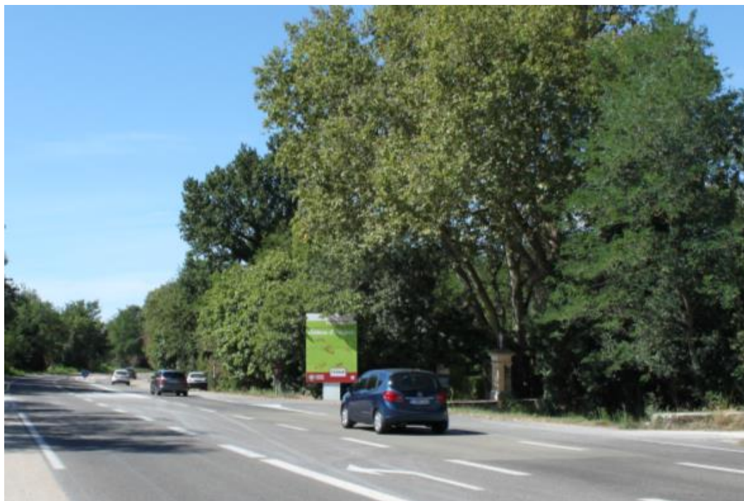
Figure 12 - An audible warning system installed on a site with a high number of bats crossings over a 37m long road section on the regional road RD530 in France. When cars are passing patches with special porous asphalt (light patch under the blue car on the picture) a high frequency sound is generated to warn bats (Photo by M. Elmeros).
