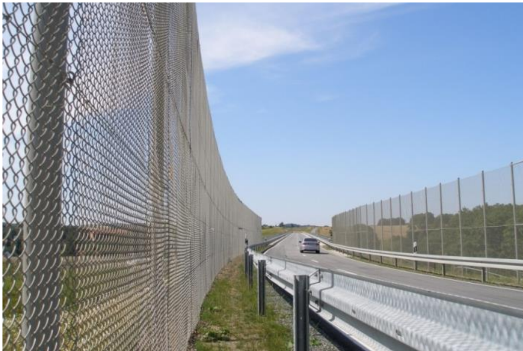
Figure 14 - Long and high fences are needed to prevent bats access to the road surface and to guide bats to safe crossing sites. The illustrated fences are installed near underpasses on the state road S170n in Germany (Photo by SWILD & NACHTaktiv).
