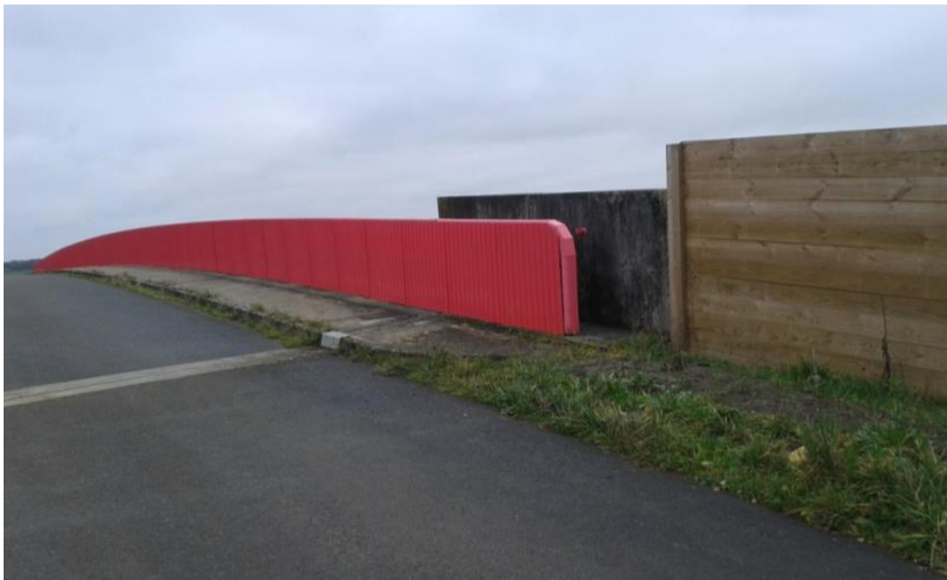
Figure 6 - Retro-fitted panels to the railings on an overbridge have increased the number of Rhinolophus bats that commuted along an overbridge in Bourges in France (Photo by L. Arthur).
