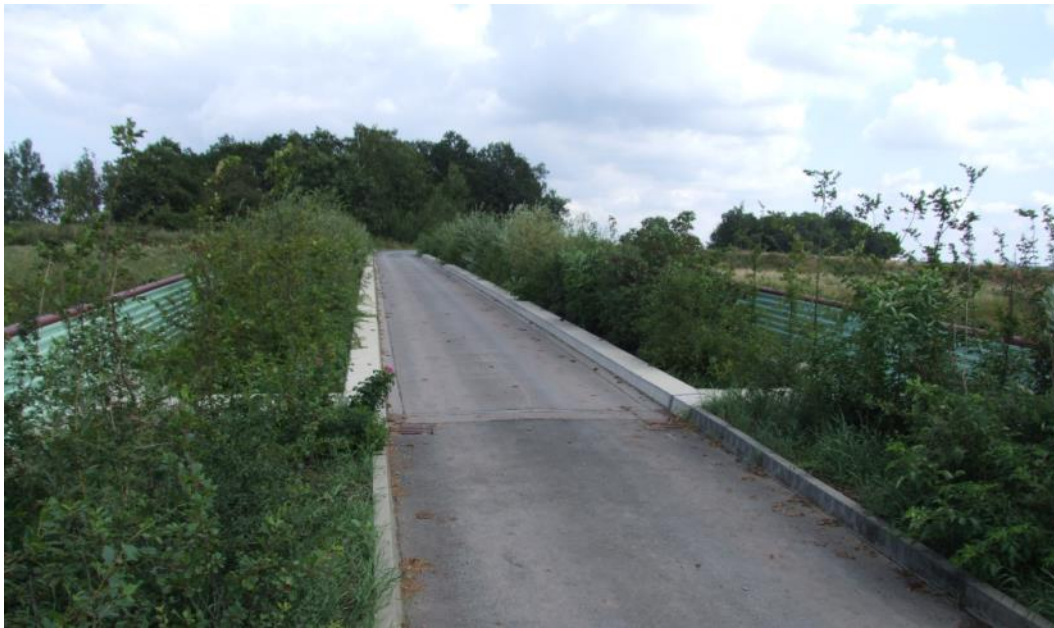
Figure 5 - A modified road overbridge with hedgerows on the state road S170n in Germany. The vegetation is to develop further to provide a dense guidance structure. Screens on the side of the overbridge provide protection of light and noise disturbance from the vehicles on the road below (Photo by SWILD & NACHTaktiv).
