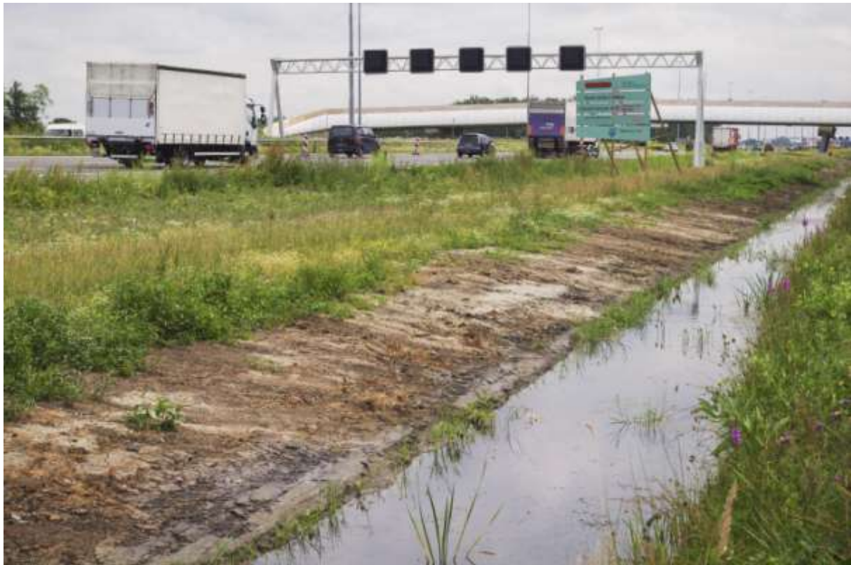
Figure 13 – A new design of roadside ditches (with a gentle slope) made the maintenance easier and increased the ecological value of the ditch (photograph: Sergé Bogaerts).
