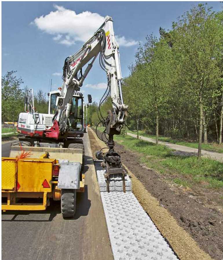
Figure 15 – To keep deer and wild boar away from the carriageway, concrete blocks with holes are placed in the first metres beside the carriageway. Grass will grow through the holes, but the concrete is not nice to walk on or dig in and therefore deer and wild boar will avoid the proximity of the carriageway. In addition, de-icing salt will not spread to the verge, but will sink through the holes directly into the ground
