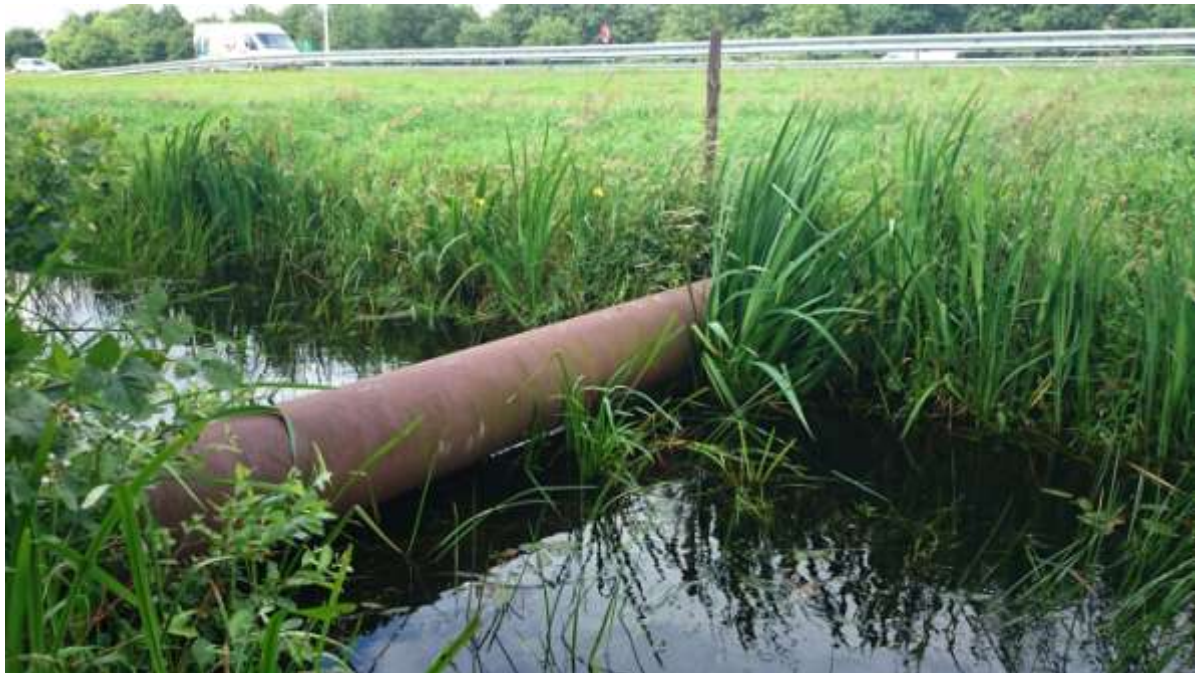
Figure 4-2 A badger tunnel made of a drainage pipe used by Badgers ( Meles meles ) to cross a highway in the Netherlands (Photograph Floris Brekelmans).
