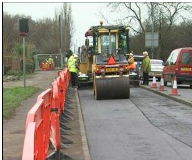
Figure 5-2 Laying of asphalt material including fly ash in Staffordshire, UK (Photo taken from Sear & Kennedy, 2010)
