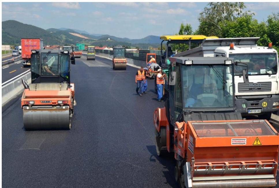
Figure 5: Rollers at paving stage – 18th May 2015
