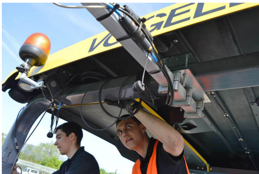
Figure 2: Mounting of the equipment on paver
