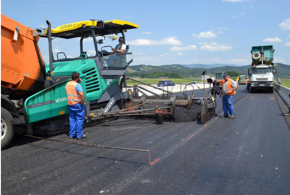
Figure 4: Echelon paving – 18th May 2015
