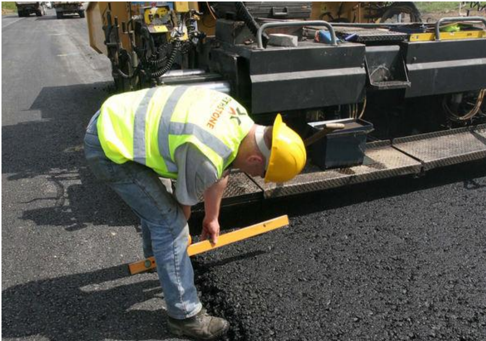
Figure 8. Layer thickness can be measured at the edge of the layer.
