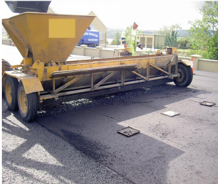
(a) HRA chippings spreader with testing trays.
