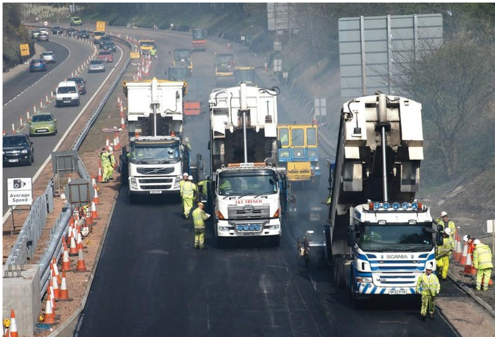
Figure 9. Echelon paving with three pavers side-by-side (www.aggbusiness.com).
