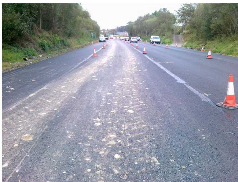
Figure 7. Example of contamination of underlying layer.
