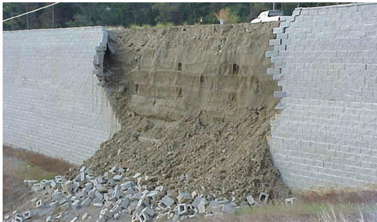
**Figure 4. Retaining wall failure.**
