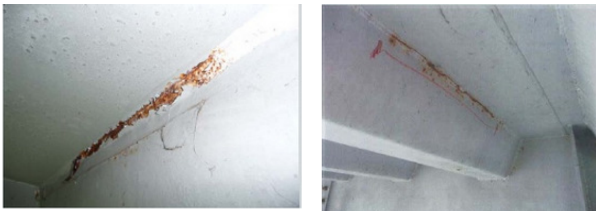
Figure 23. Cracks at the weld between the steel deck and the longitudinal stiffener.
