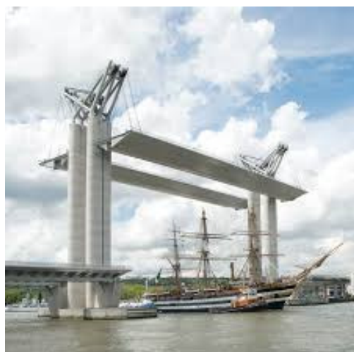
Figure 22. Moveable bridge of Rouen, with orthotropic deck.
