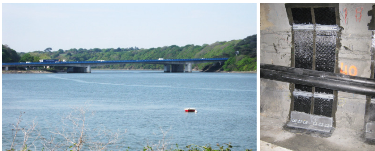
Figure 26. Bridge near Scorff (Lorient). Transverse strengthening of a bridge which is longitudinally prestressed.
