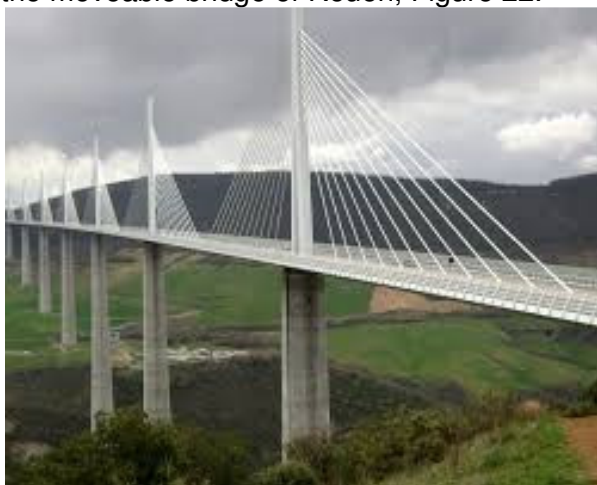
Figure 21. Cable-stayed Millau viaduct, whose deck is orthotropic.
