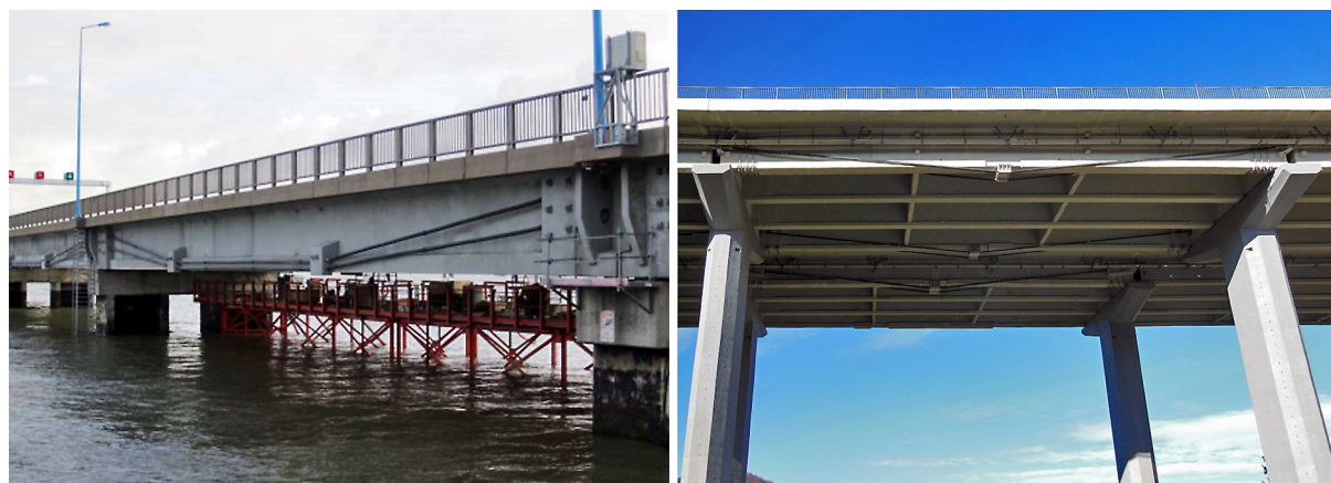
Figure 27. Additional prestressing on the Saint Nazaire bridge (France) and Ravbarkomanda bridge (Slovenia).
