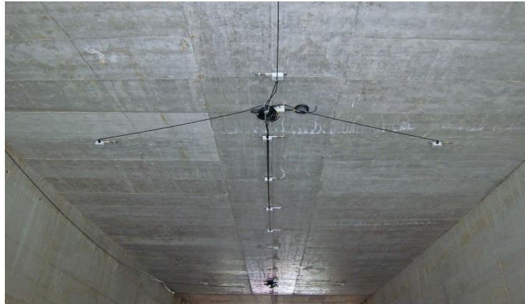
Figure 7: Bridge instrumentation with strain transducers
