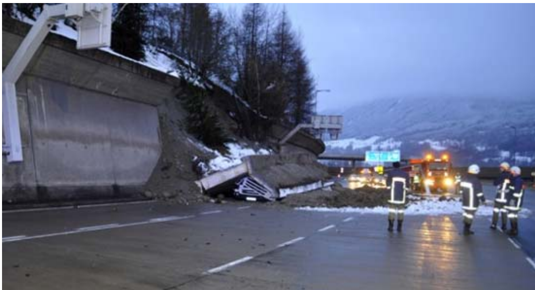
Figure 2.1 Wall failure in Austria (OE24, 2012)
