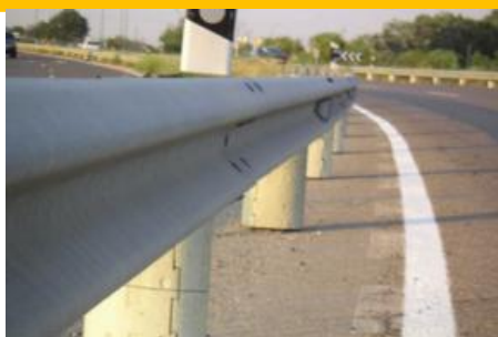
Figure 76 - PVC foam made impact attenuators for bollards Photo by (Vieira et al. 2008)
