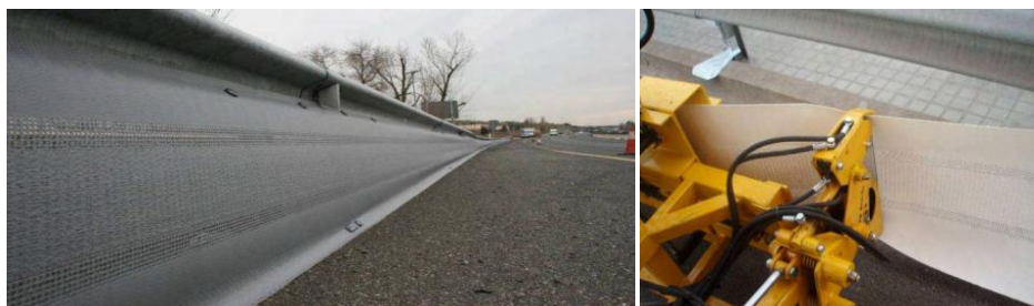
Figure 75 - New, innovative protection system BASYC: special impact attenuator mesh used for personal vehicles and motorcyclists collision protection. Photo by (Sistemas de Seguridad Vial)
