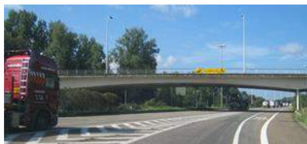
Figure 38: A21/E34 - Road work signing scheme
