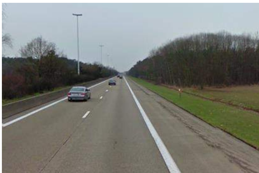
Figure 35: View of the A21/E34 (between Zoersel & Oelegem) before the 2014 works (structure rehabilitation)
