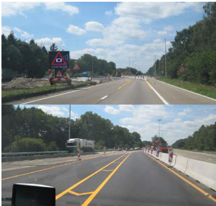
Figure 87: 2014 Road works along the A21/E34 Belgian motorway: longer transition, softer deviation angle in the crossover
