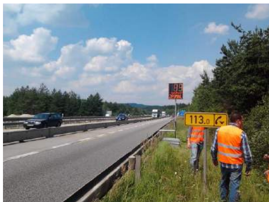
Figure 10: View of the temporary crash barrier used to separate opposite traffic flows
