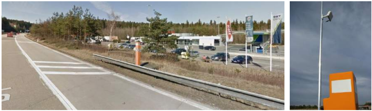
Figure 14: Overview of the detection site n°2
