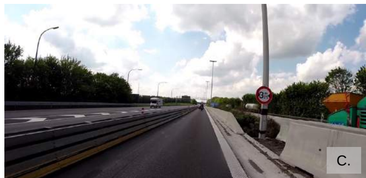
Figure 26: Temporary traffic management around the transition area (work area = green area) during the second stage of the works
