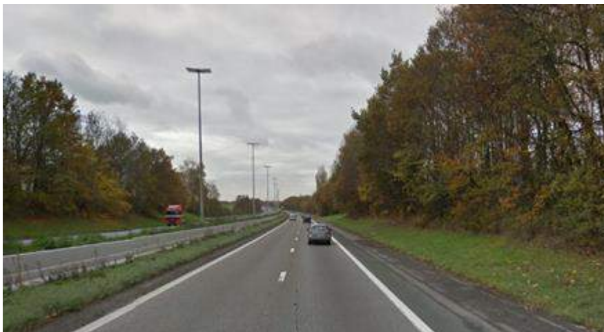
Figure 25: View of the A15/E42 (between Daussoulx & Sambreville) before the 2014 works (additional lane to be built on the left side and new pavement to be laid across all the lanes)
