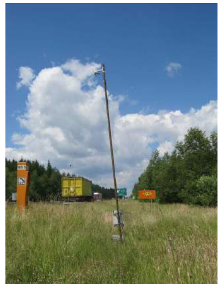
Figure 15: Overview of the detection site n°3 and installation of the Wavetronix detector
