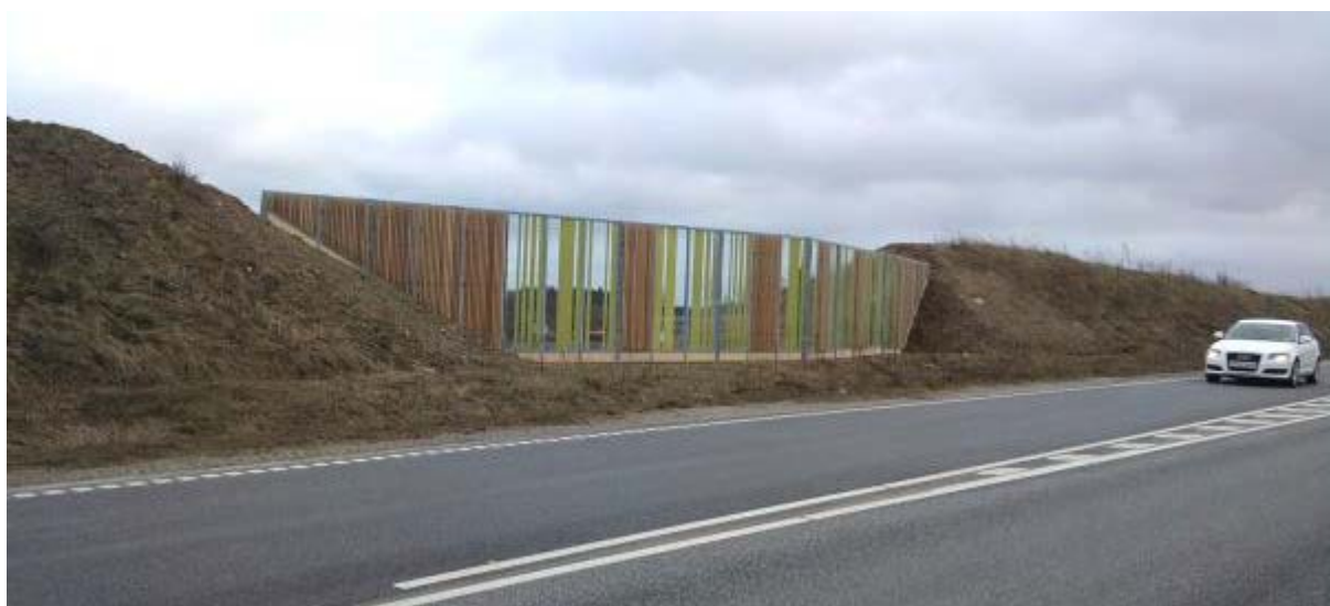
Figure 5.13: New residential area constructed along an existing main road. As part of the project, the developer has constructed and financed a combination of noise barriers and earth walls.
