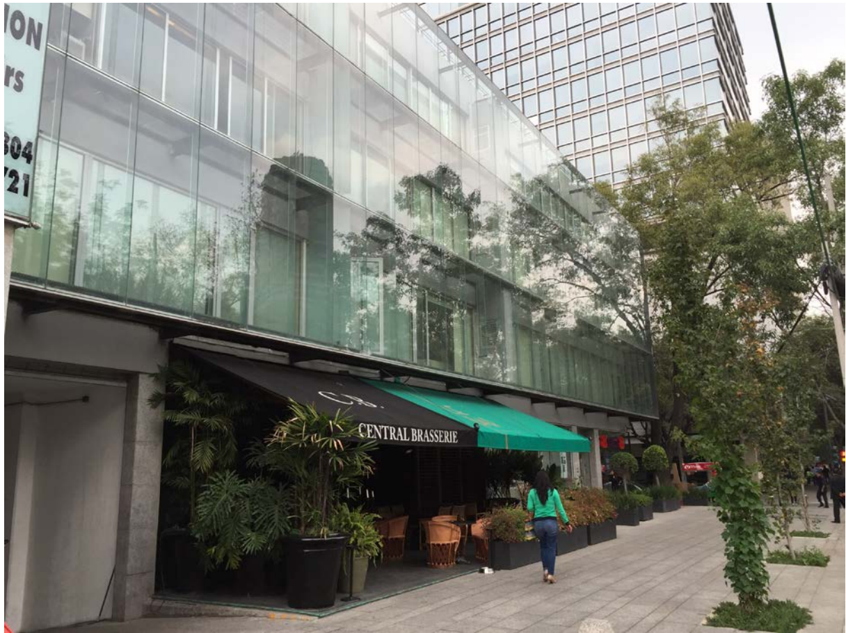
Figure 3.20: New glass façade in front of the existing façade at residential building in Mexico City.
