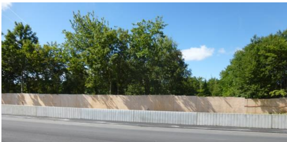
Figure 6.3: Temporary 2 m high noise barrier of plywood panels along highway enlargement project. After the construction work, it was replaced by a permanent noise barrier. The low concrete wall in the front is the foundation of the permanent noise barrier.
