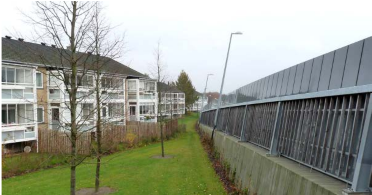
Figure 4.14: Balconies covered by glass in order to reduce noise from a nearby highway, as the noise barrier did not provide sufficient noise reduction to fulfil noise limits.
