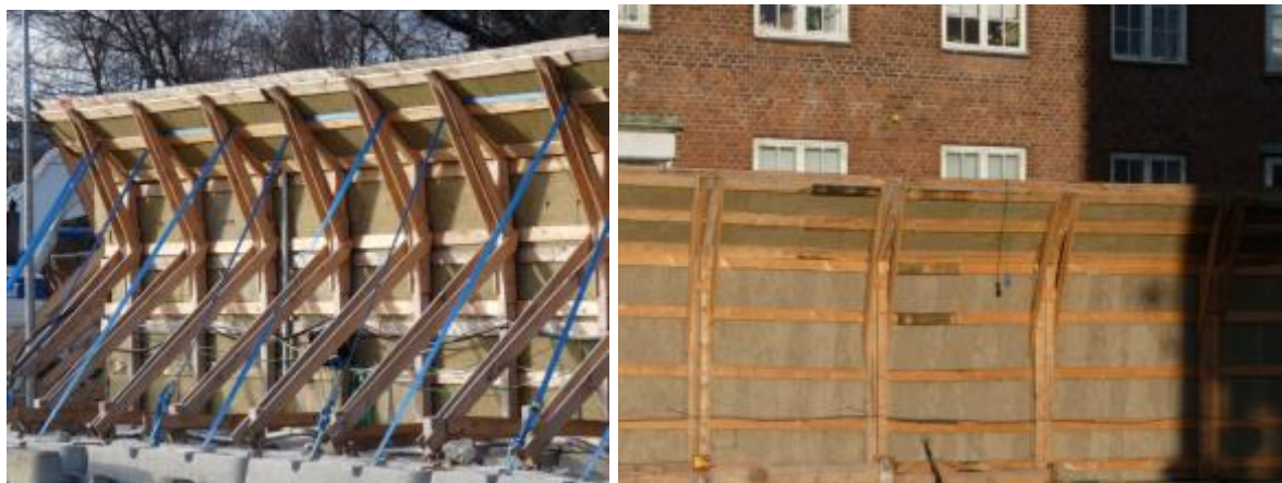
Figure 6.4: Temporary 4 m high wooden noise barrier with absorbing and noise-reducing mineral wool at the construction side of the barrier. The barrier is bending towards the construction site to increase the noise reduction.
