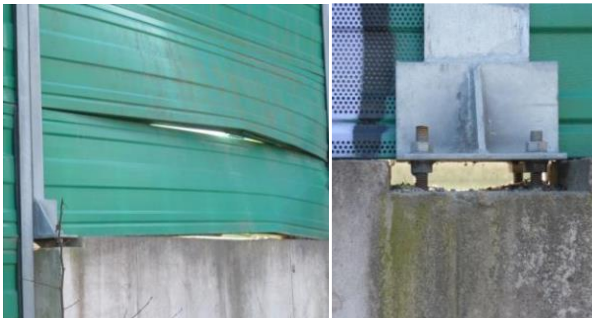
Figure 5.5: Steel noise barrier damaged by snow removal equipment (left). The two open cracks reduce the acoustic effect. The opening between the steel post and concrete foundation (right) also reduces the acoustic effect.
