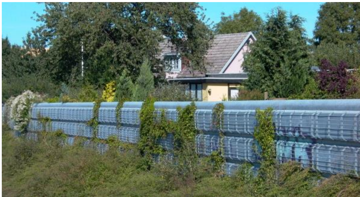
Figure 5.7: Noise barriers with vegetation which might need maintenance of the vegetation.
