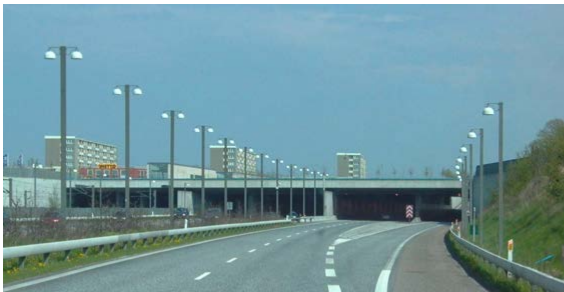
Figure 4.12: A new highway near the Copenhagen airport covered at a section of 700 m where the highway passes some blocks of apartments. The areas over the highway have
