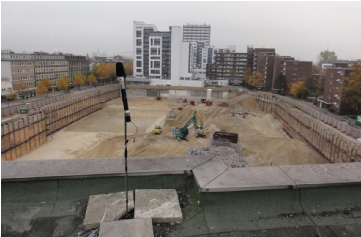
Figure 6.8: Continuous noise monitoring systems overlooking the IKEA construction site in Hamburg, Germany.
