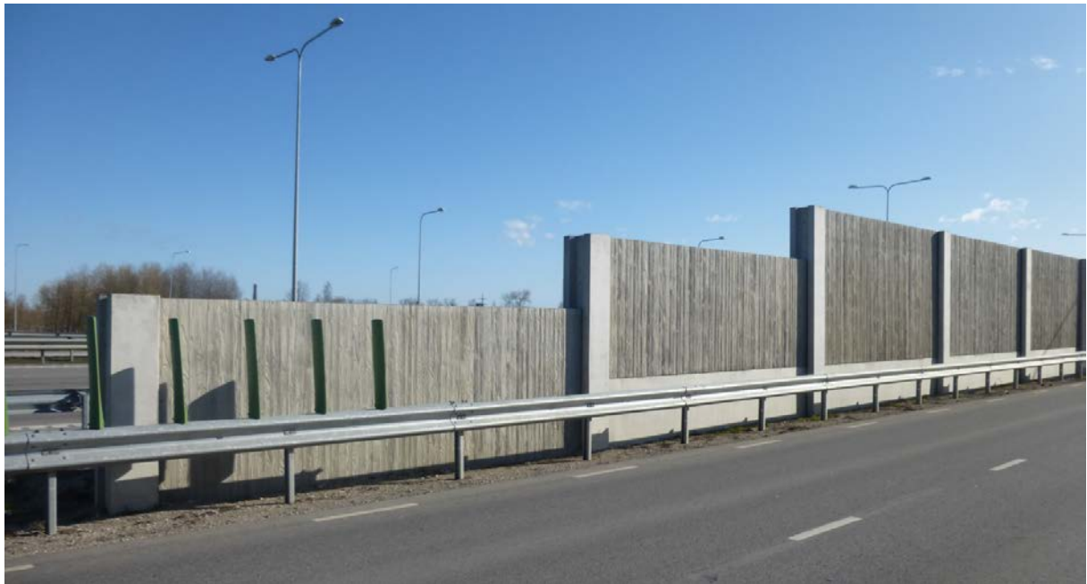
Figure 5.10: Noise barrier of structured concrete constructed by the road administration along an existing highway in Tallinn, Estonia to protect an area with villas.
