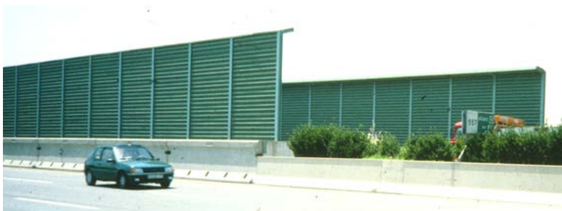
Figure 3.17: High noise barriers placed both at the side of a highway and at the centre of the highway in order to increase the noise reducing effect on a highway in Italy.
