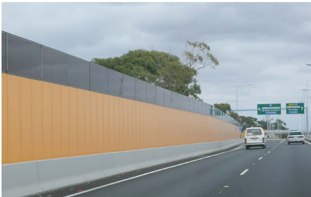
Figure 4.13: Noise barrier with vertical photovoltaic panels at the top (by permission of VicRoads, Melbourne, Australia).
