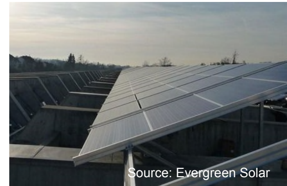
Noise-protection tunnel with a solar power plant on the roof, highway A3 near Aschaffenburg, Germany
