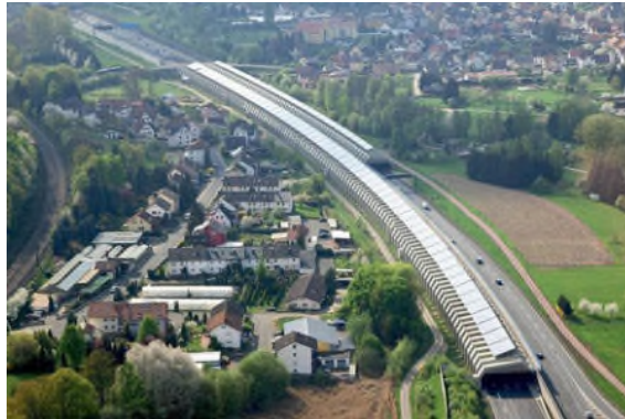
Noise-protection tunnel with a solar power plant on the roof, highway A3 near Aschaffenburg, Germany
