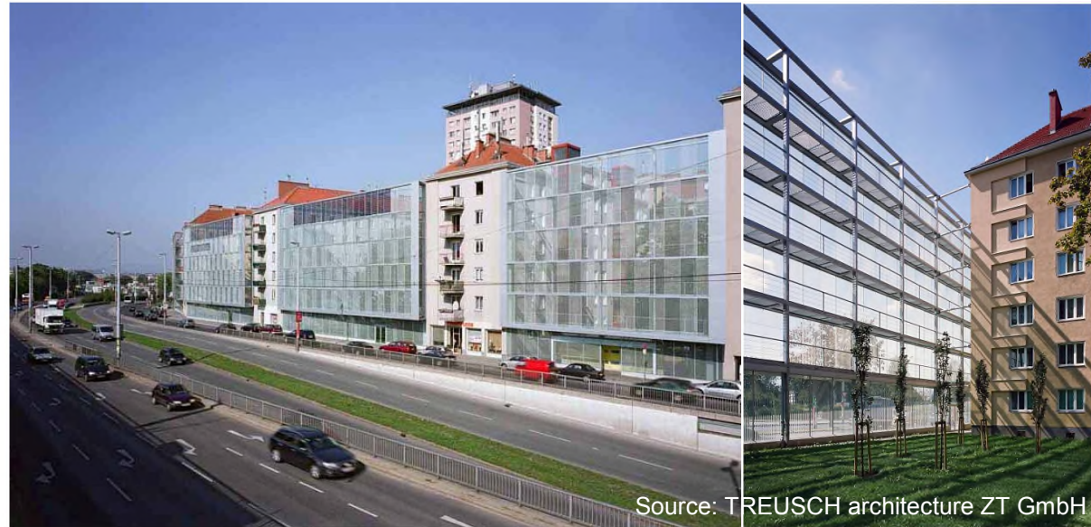
Glass noise screen at the Theodor-Körner-Hof: street (left) and courtyard view (right)
