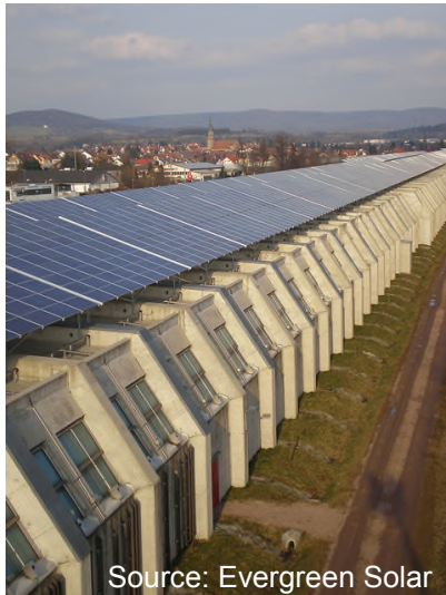
Detail of a noise-protection tunnel with solar panels, Aschaffenburg, Germany
