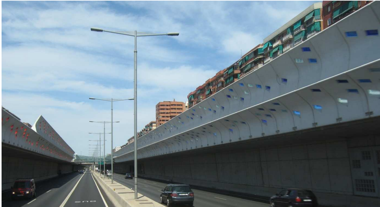
Figure 5.4: Motorway in a trench with high noise barriers on each side to provide noise protection to nearby blocks of flats.
