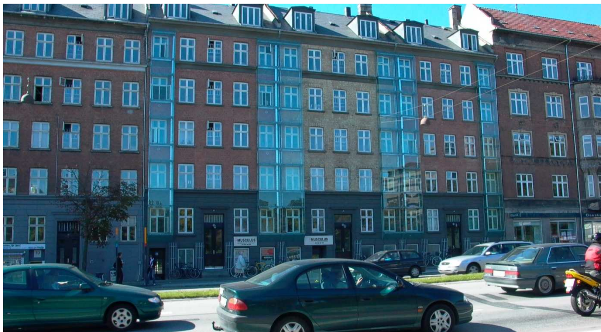
Figure 5.6: A noise insulation glass enclosure has been placed in front of the living room windows in this block of flats along a main urban road where there is no space for constructing noise barriers.
