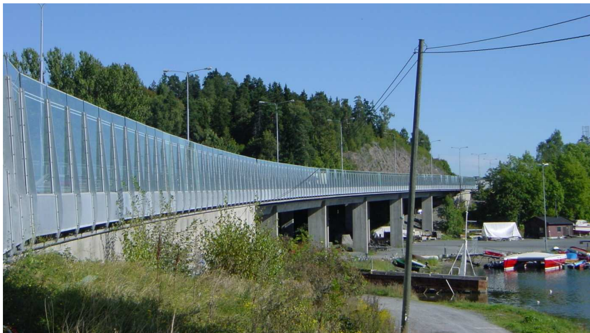
Figure 3.6: Glass noise barrier outside Oslo, Norway. Source: Norwegian Public Road Administration, 2008.
