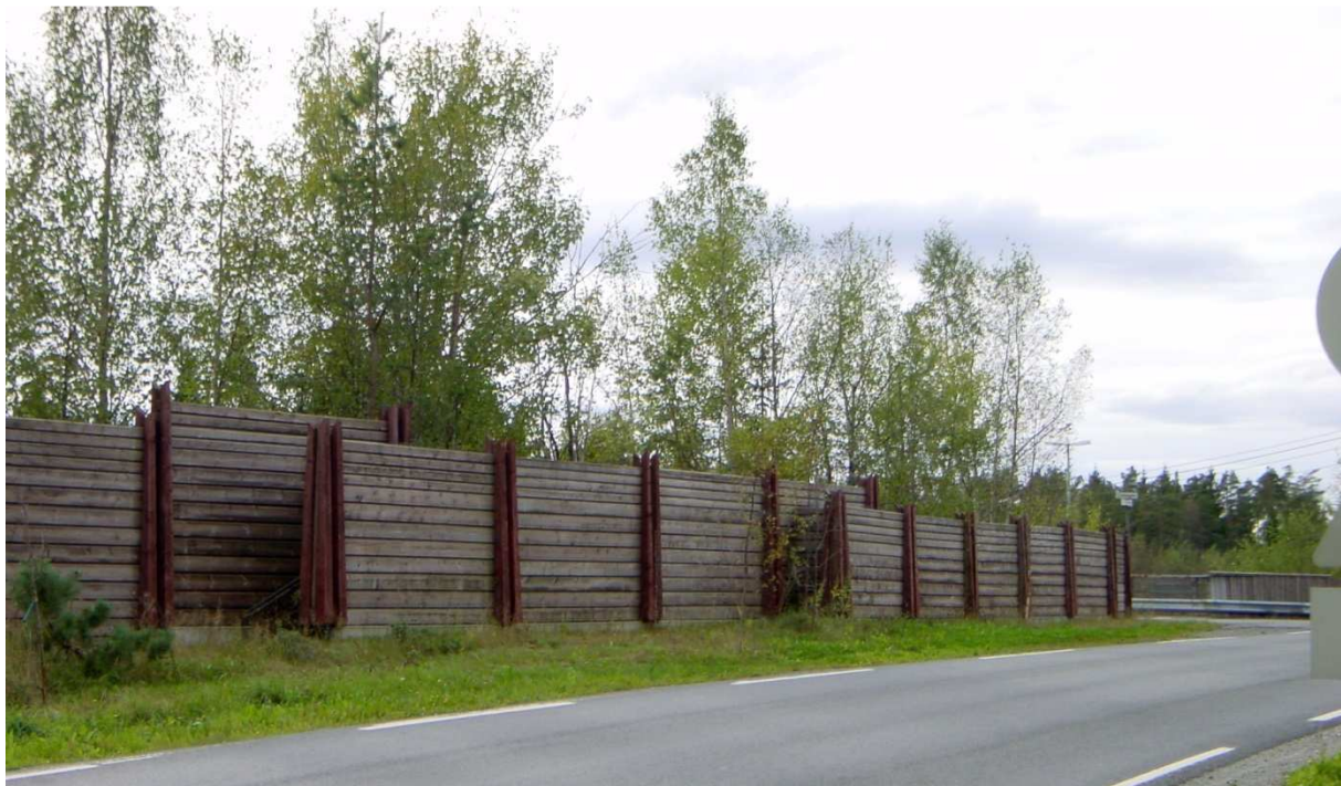
Figure 3.3: Noise barrier in Asker, Norway. Source: Norwegian Public Road Administration, 2008.
