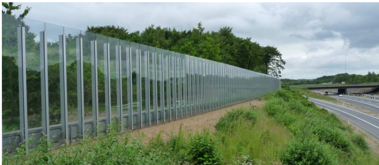
Figure 5.2: Transparent noise barrier along motorway.
