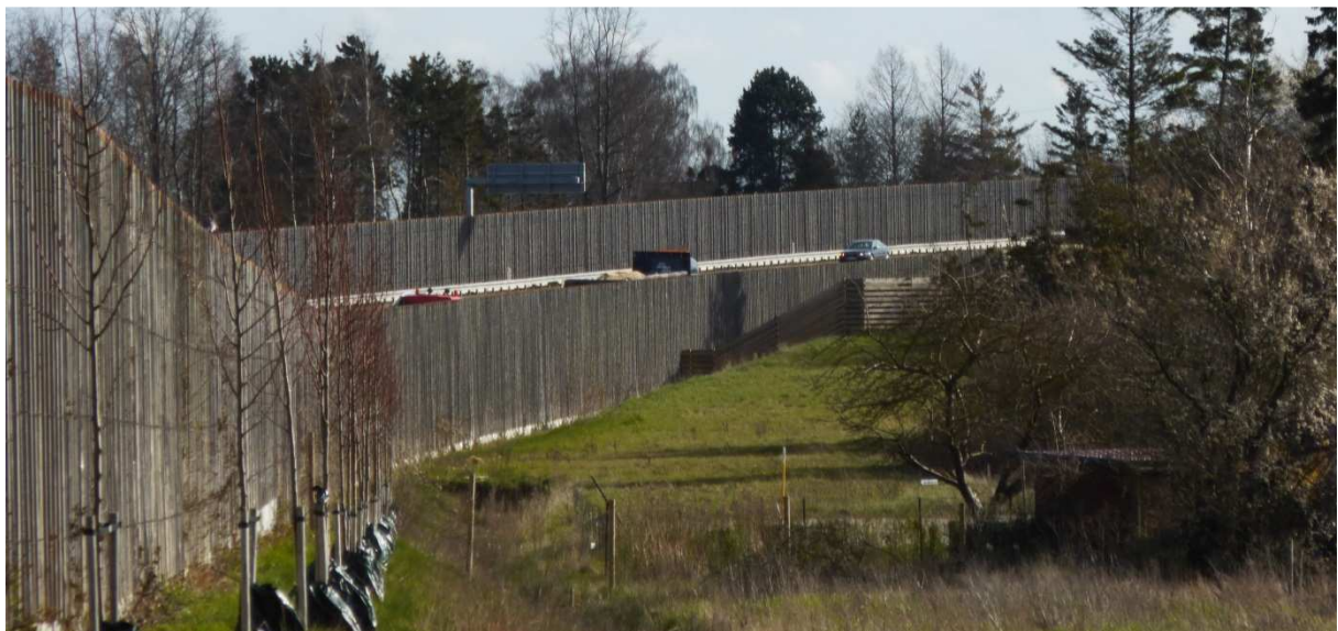
Figure 5.1: Long wooden noise barriers along both sides of a motorway protecting nearby residential areas.
