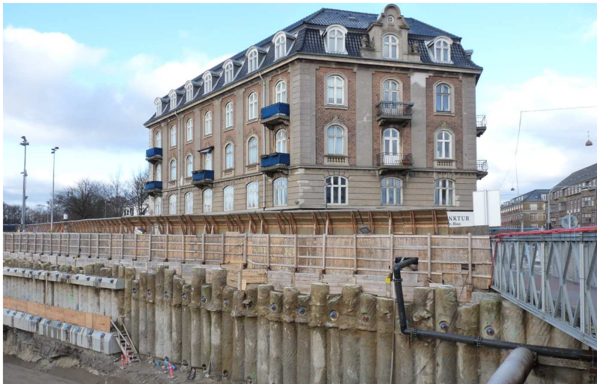
Figure 3.5: Temporary wooden noise barriers built around a new road construction site.
