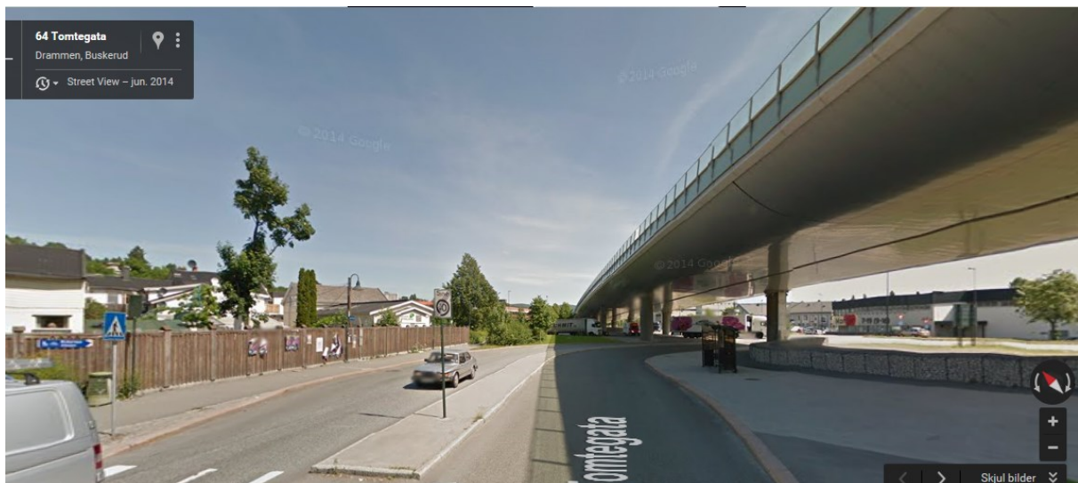
Figure 30: Residential area northwest of the flyover seen from the local road; from Google Street view 2014
