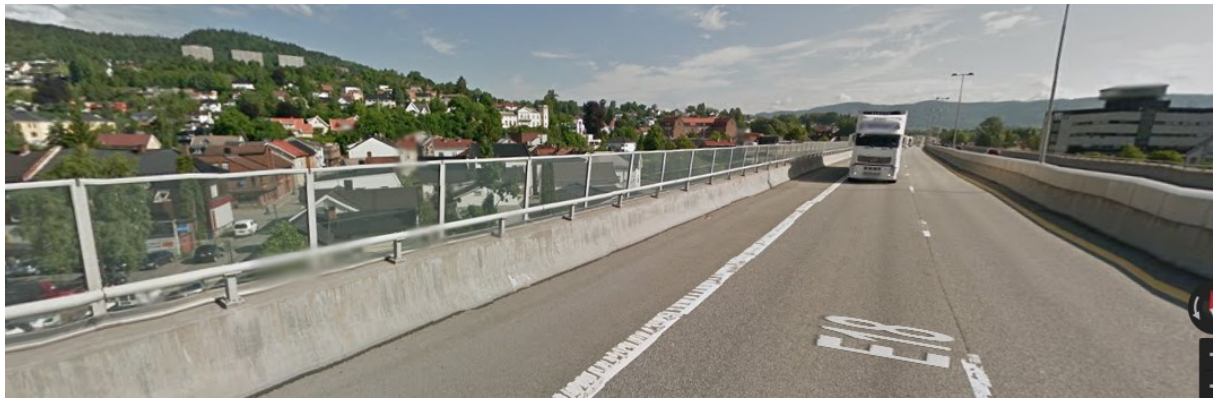
Figure 29: Residential area northwest of the flyover seen from the motorway flyover; from Google Street view 2014
