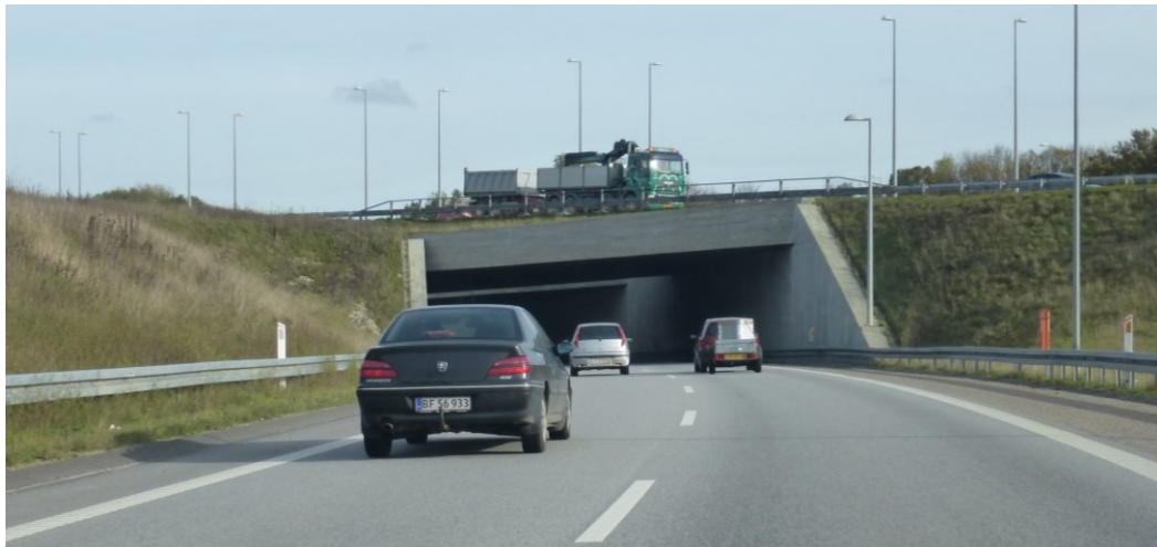
Figure 23: Eastbound lanes of M12 passing under M3
