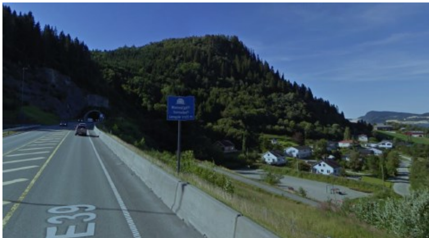
Figure 20: Mannsfjell-tunnel opening and surrounding terrain. From Google Streetview, 2010
