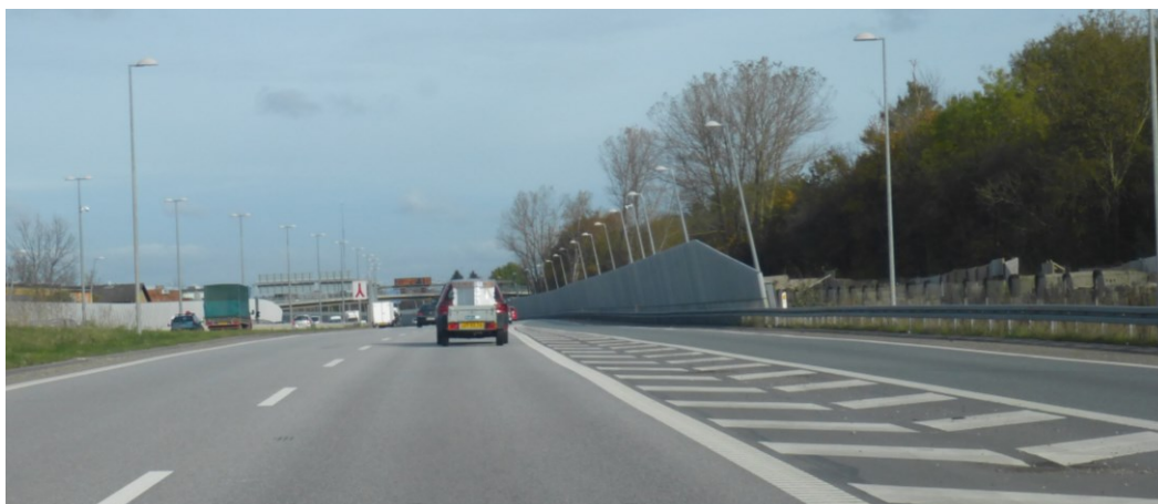
Figure 25: Northbound lanes of M3 with noise barrier where M12 joins M3 north of Jyllingevej
