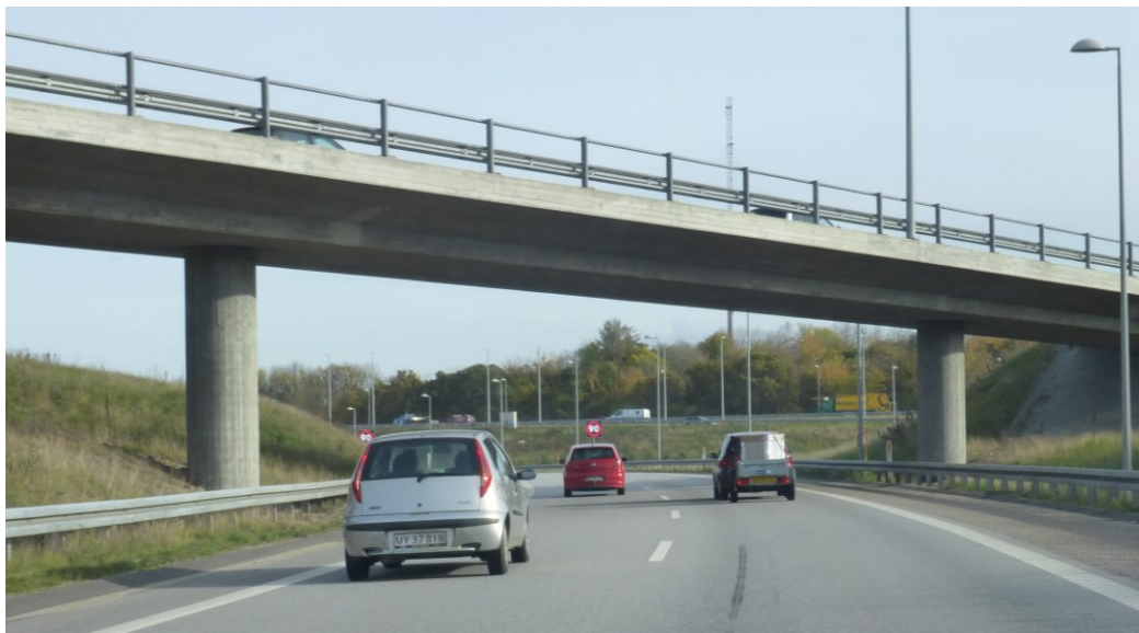
Figure 24: Eastbound lanes of M12 passing under westbound lanes of M12
