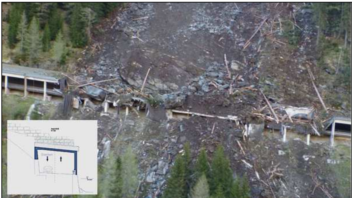
Figure 5: The Felbertauernstraße in May 2013, hit by a landslide. In this context it was said that half-tunnels might work as an adaption measure. A total relocation, abandoning the road is only an option if there are other ways to guarantee the supply of remote regions.
