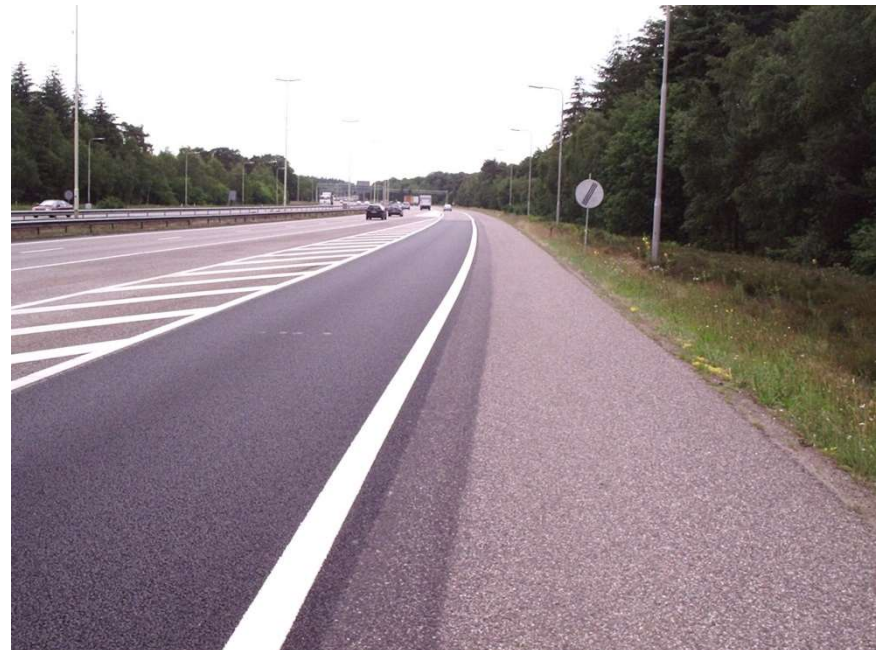
Spay emulsion bitumen with rejuvenators
