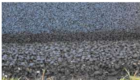
Figure 1: Example of two-layer porous asphalt
