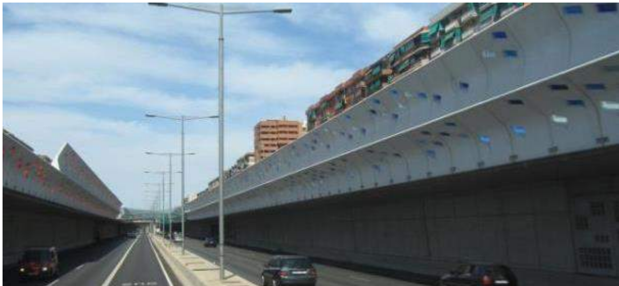
Figure 4.10: Highway through a densely populated area in Barcelona, Spain, constructed in a ditch with concrete sides and noise barriers bending over the road.
