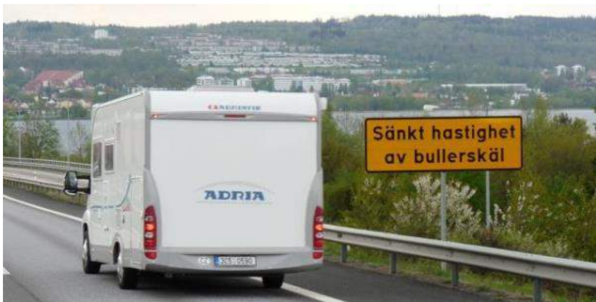
Figure 4.16: A speed reduction from 110 to 90km/h was part of a noise reduction project along 3km of Highway E4 passing a residential area near Husqvarna, Sweden, with a traffic volume of 22,000 vehicles per day. The sign at the roadside states 'Reduced speed because of noise' (refer to example in Annex C for more details).
