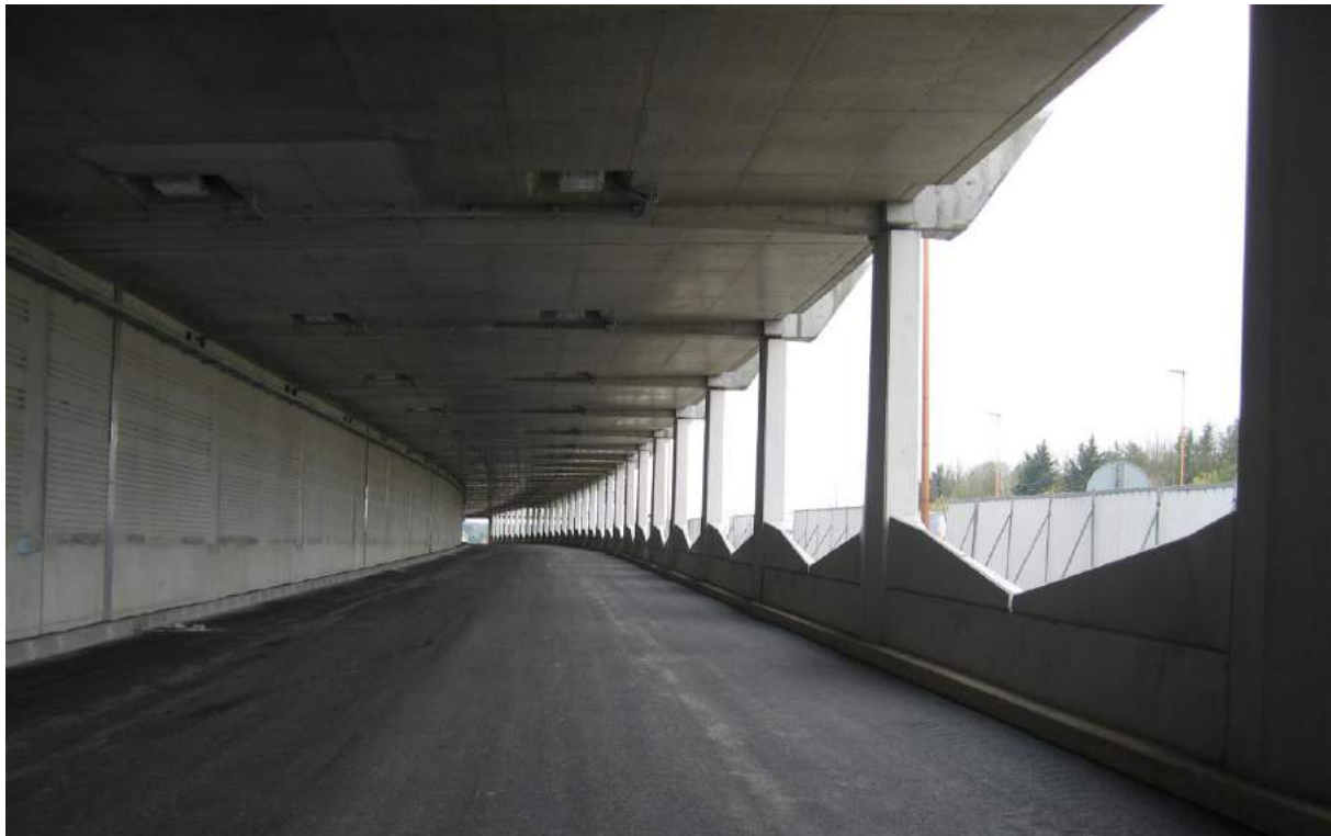
Figure 4.2: According to the principles of sustainability, the network's environmental footprint should be kept to a minimum. This often requires huge investments in noise abatement as part of new highway projects. The image shows the partial covering of a motorway in Paris.
