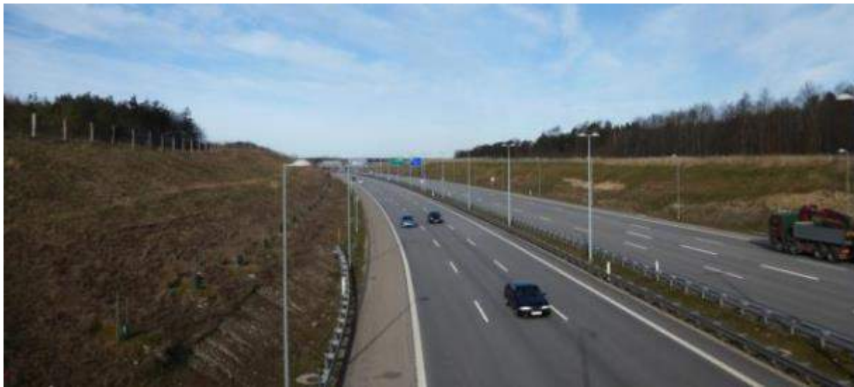
Figure 4.9: A new highway in Denmark constructed in a ditch with an earth wall at the side. The sides of the ditch, which include vegetation, are noise absorbing.
