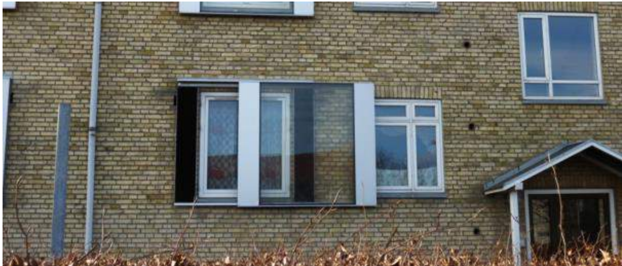
Figure 5.9: Publicly financed movable noise protection (noise shutters) placed in front of an existing living room window on a residential building along an arterial road in Copenhagen.
