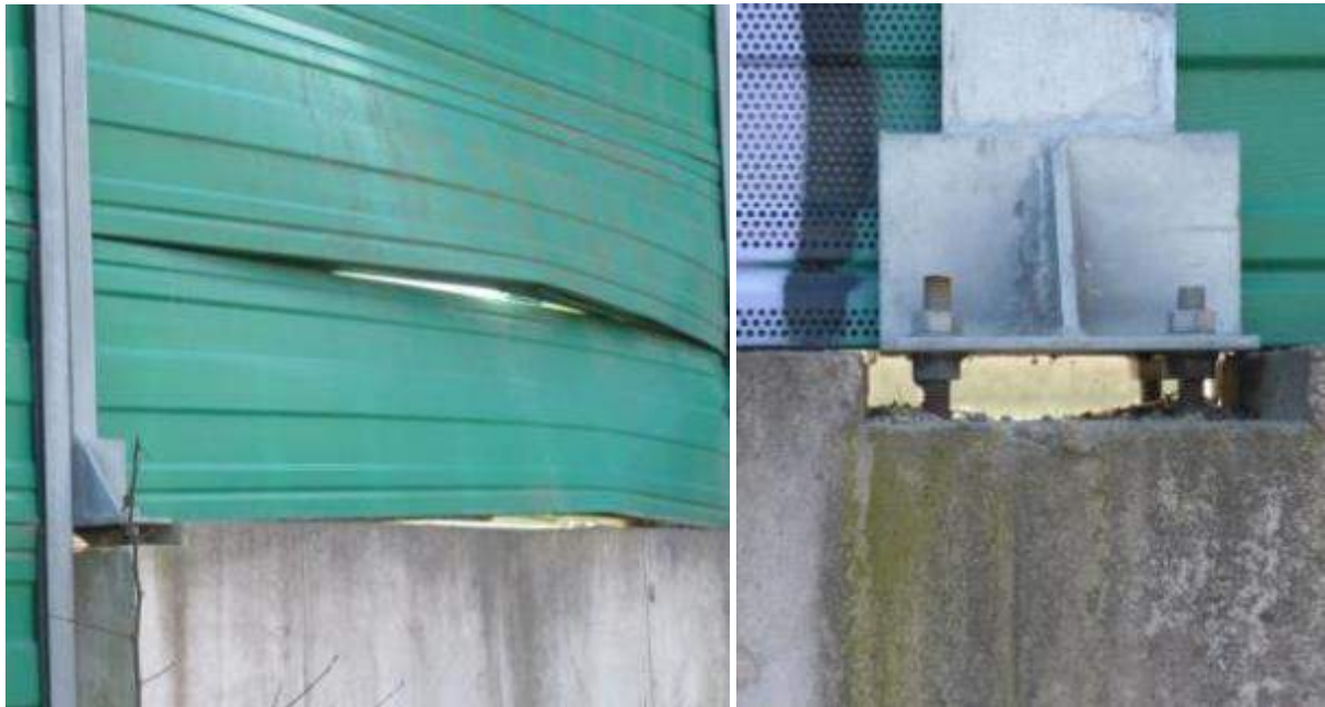
Figure 5.5: Steel noise barrier damaged by snow removal equipment (left). The two open cracks reduce the acoustic effect. The opening between the steel post and concrete foundation (right) also reduces the acoustic effect.
