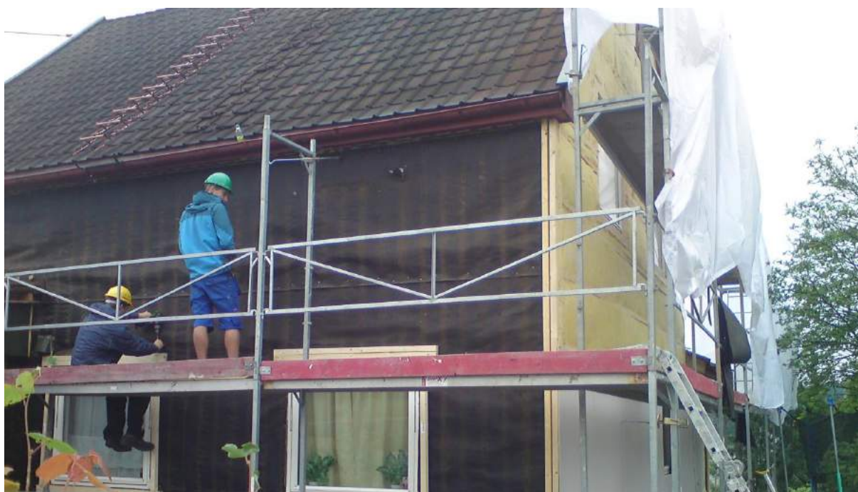
Figure 5.11: Façade insulation of dwellings along existing highway in Norway, financed by the road administration (photo by the Norwegian Public Roads Administration).
