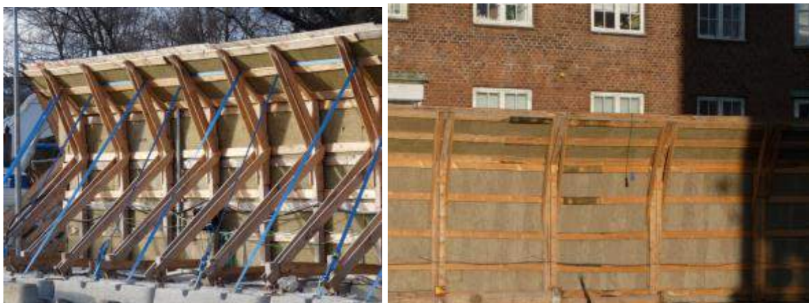
Figure 6.3: Temporary 2m high noise barrier of plywood panels along highway enlargement project. After the construction work, it was replaced by a permanent noise barrier. The low concrete wall in the front is the foundation of the permanent noise barrier.
