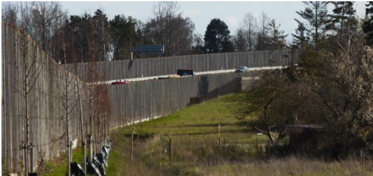
Figure 3.15: Long steel noise barriers with wooden slants along both sides of a motorway, protecting nearby residential areas.
