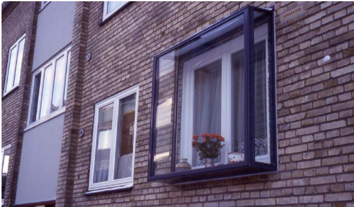
Figure 3.18: Extra noise protection as a glass box placed in front of existing living room window. No noise protection has been applied to the kitchen window to the left.
