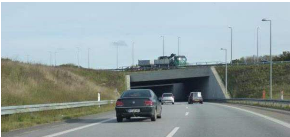
Figure 4.11: The ramp of a highway intersection, constructed as a 'flyunder' to reduce noise exposure to neighbouring residential and public green areas.
