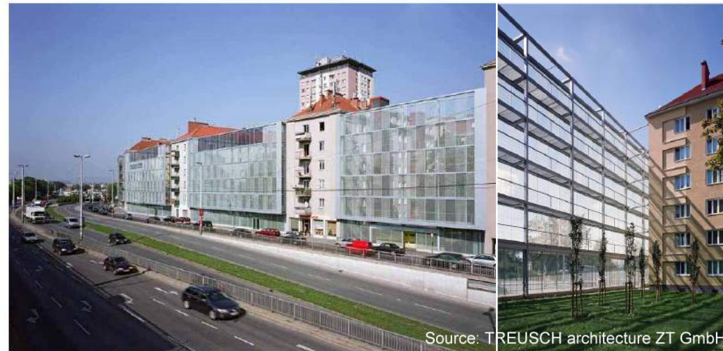
Glass noise screen at the Theodor-Körner-Hof: street (left) and courtyard view (right)
