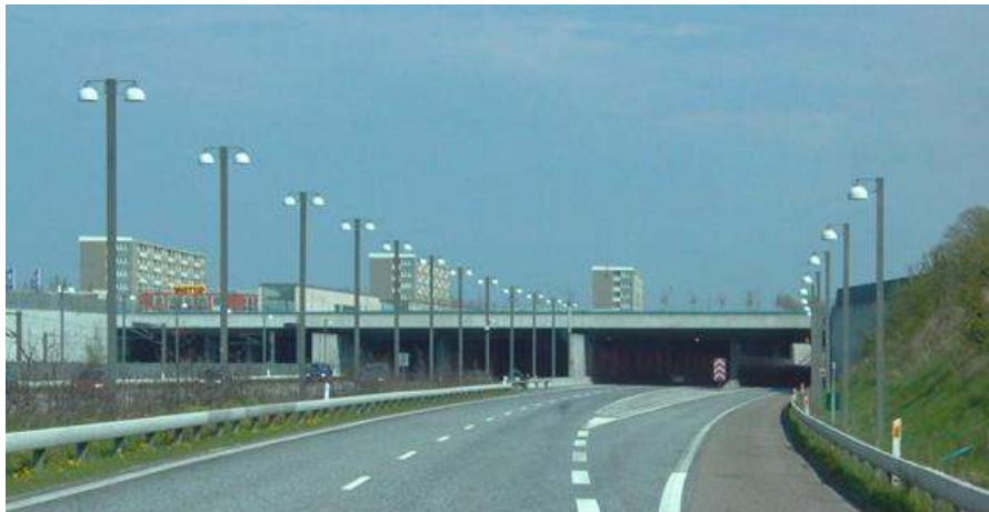
Figure 4.12: A new highway near the Copenhagen airport covered at a section of 700m where the highway passes some blocks of apartments. The areas over the highway have been used as a green area, binding the urban environment at the two sides of the highway together.
