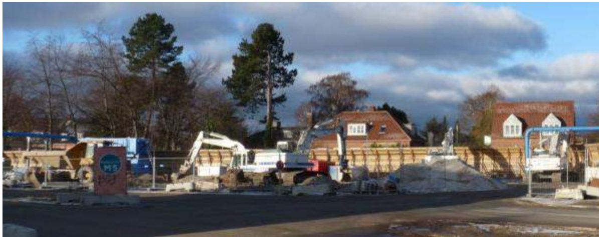
Figure 6.2: A given excavator has a certain noise emission level. The total noise contribution from this machine also depends on the number of machines used, the duration of the working process, the time of the day and the distance to noise receiver points.
