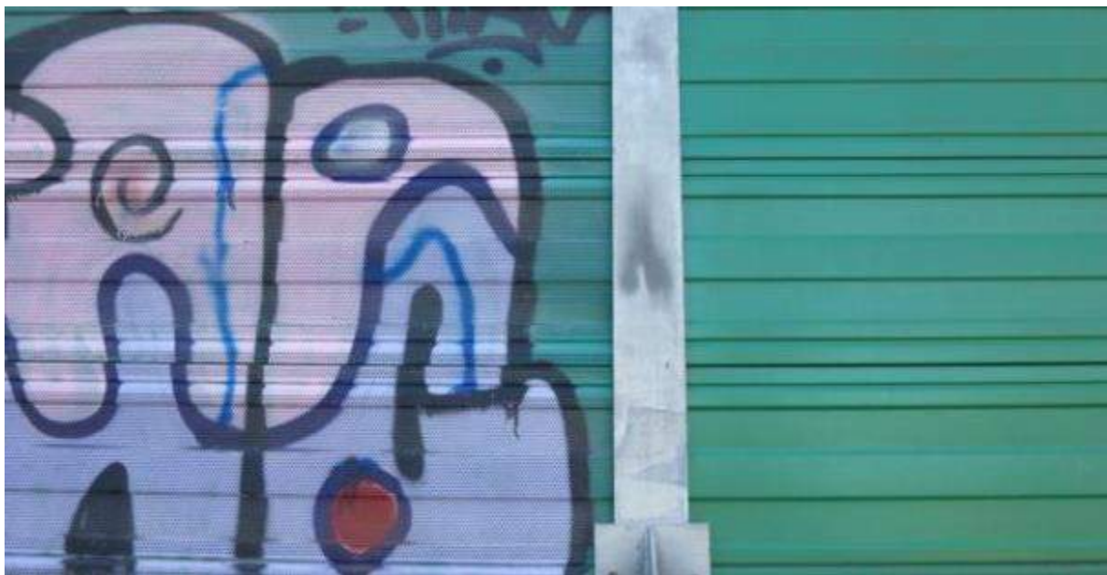
Figure 5.4: At some locations, graffiti can be a problem which detracts from the visual appearance of noise barriers. Cleaning activities are needed in such situations.
