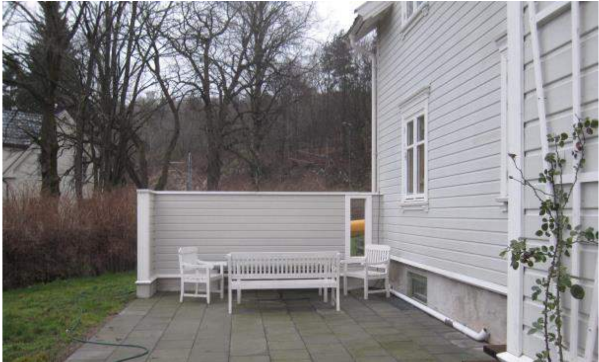
Figure 4.15: A single house in Norway with local white wooden noise barrier around the terrace designed in the same style as the house (photo by permission from the Norwegian Road Administration).
