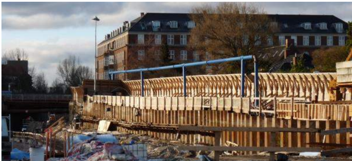
Figure 6.1: New urban highway under construction as a cut-and-cover process in densely built-up residential area in Copenhagen, Denmark. Temporary wooden noise barriers have been established to reduce the construction noise.
