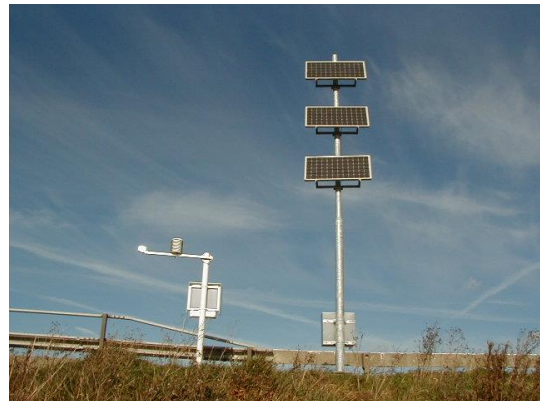
Fig. 9: A solar-powered road weather station
