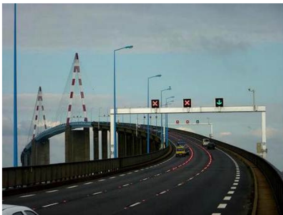
Figure 11: Dynamic lane management on a reversible lane on St Nazaire Bridge (France) (© CETE Ouest)
