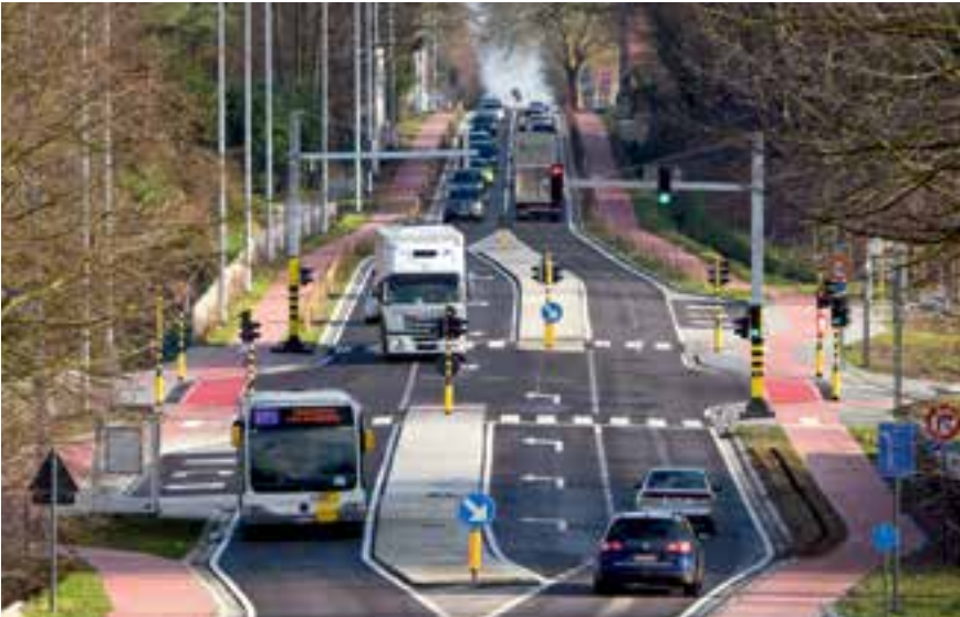
This intersection on the Brusselsesteenweg (N2) in Herent was redeveloped in 2012. Due to the wide cycle paths and narrower lanes, this reconstructed road is safer for both cyclists and motorised traffic.
