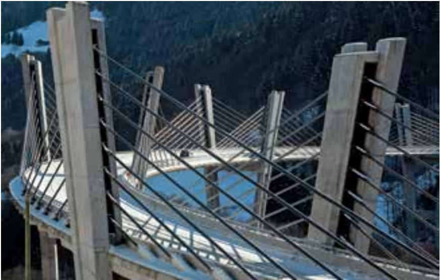
View of the Sunniberg Bridge in Klosters, a late work by the internationally renowned engineer Christian Menn. The bridge is 526 m long and has a curvature radius of around 500 m.
