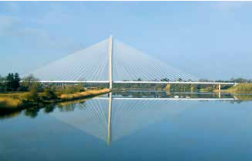
The River Suir Bridge (N25 Waterford Bypass route) has a total length of 450 m and a main span of 230 m, which is the longest road bridge span in Ireland.
