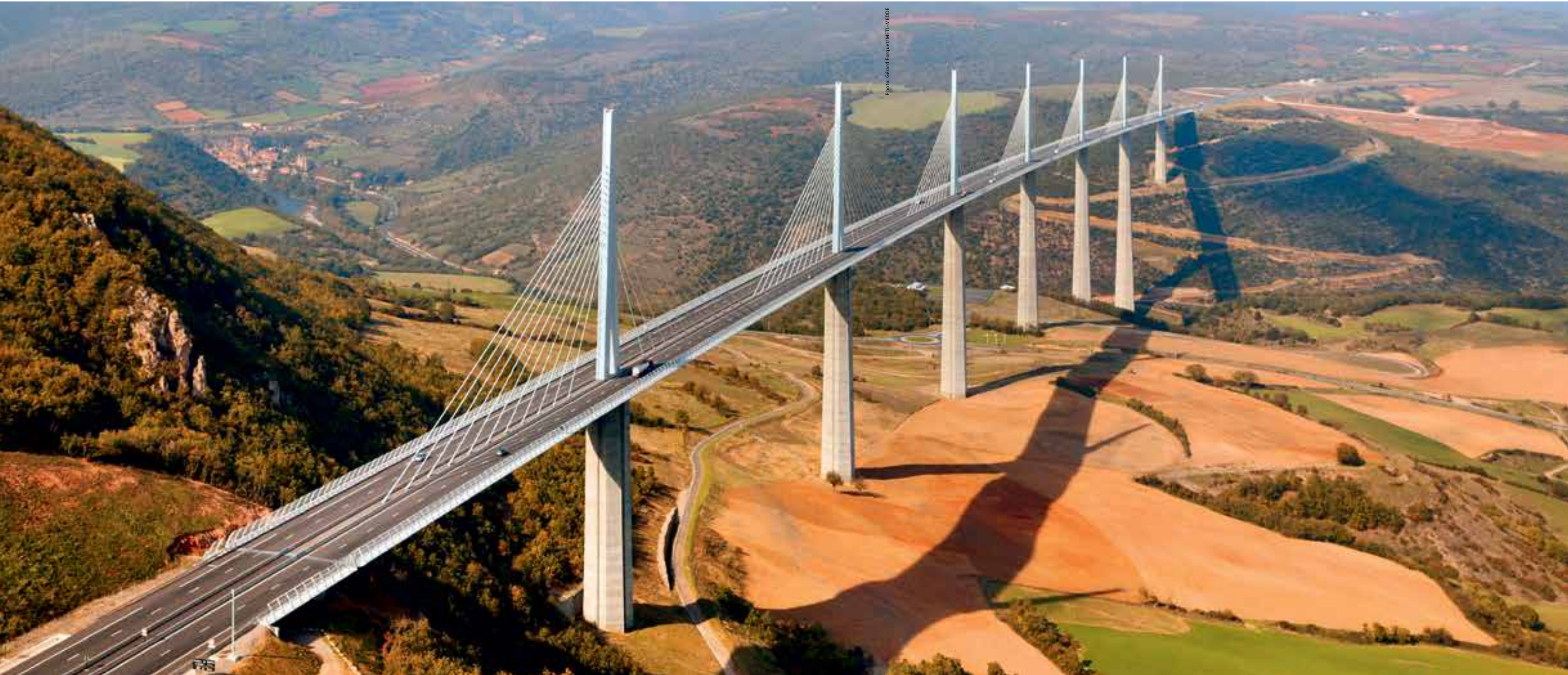
The Millau Viaduct is often described as a work of both engineering prowess and architectural grace, and has become a tourist attraction in its own right. It is part of the A75 Motorway crossing the Tarn Valley in the south of France. This road structure, the construction of which ended in 2004, set four world records at the time of its commissioning: the world's highest pier (245 m), spire (343 m) and road deck (270 m) and the world's longest cable-stayed deck (2,460 m).
