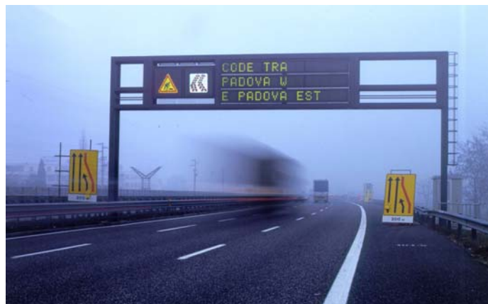
Fig. 12: Italy : the use of 2 pictograms with text (please note that 'dark and light' inversion is not used in Italy)
