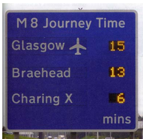
Fig. 10: This kind of sign can also provide link information and is used in Scotland and Australia
