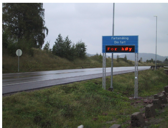
Fig. 19: Norwegian VMS that alert drivers to excessive speeds (Fartsmåling = Speed measurement; Din fart = Your speed; For høy = Too fast)
