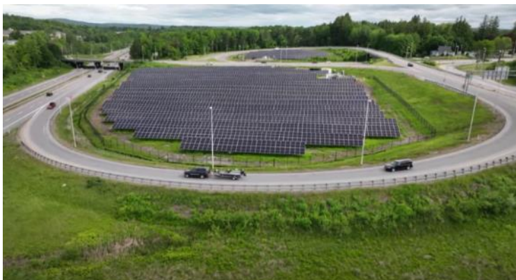
Figure 2.- Solar highway installation in Augusta, Maine, built by Maine DOT. Source: Maine DOT (2023)
