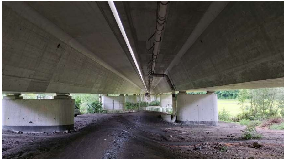
Figure 29: Multi-span highway viaduct – view from below.
