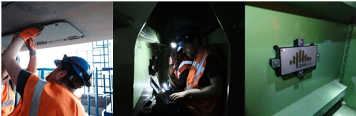
Figure 25: Installation of the sensors UniQ on the bridge.
