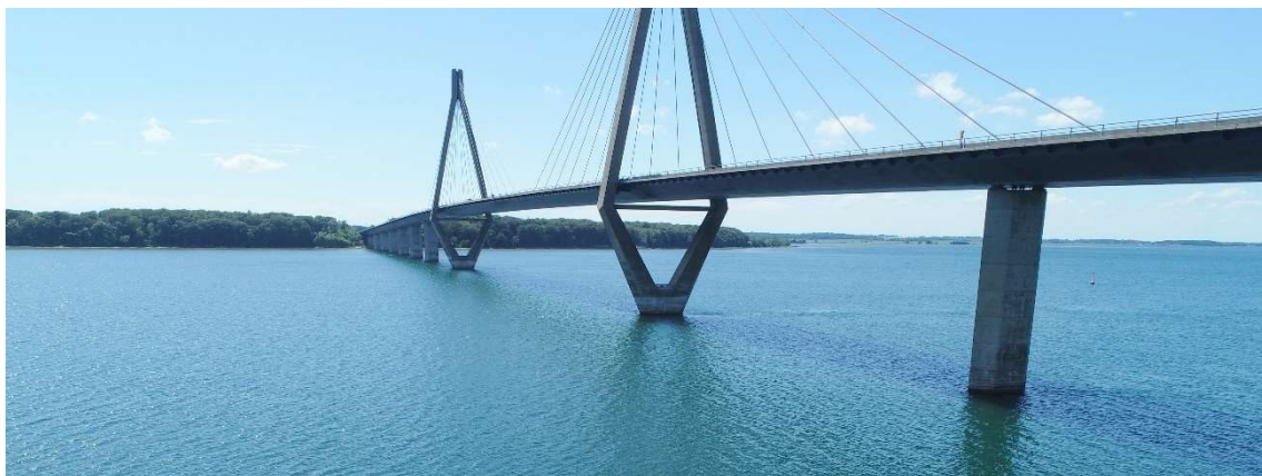
Figure 19: The Farø Bridges. Cable-stayed bridge.
