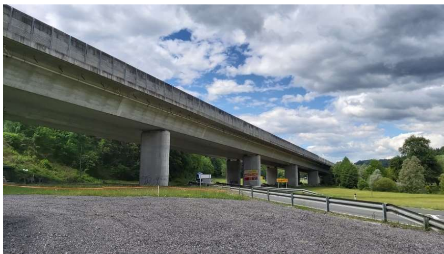
Figure 28: Multi-span highway viaduct – side view.
