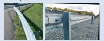
Description: Safety barrier made of steel. Semi-rigid barriers, usually made from steel beams or rails. Most common type is the W-Beam steel barrier.
