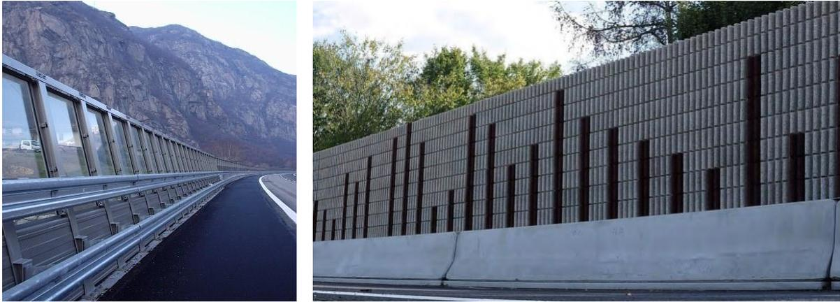
Figure 2: Different types of integrated noise and safety barriers of different materials in Europe (steel & transparent left side and fully concrete type right side).
