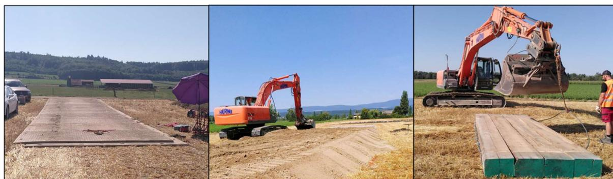
**Figure 3.** The access materials employed. From left to right: composite mats, sand track and wooden mattress. Photos by Loraine ten Damme.
