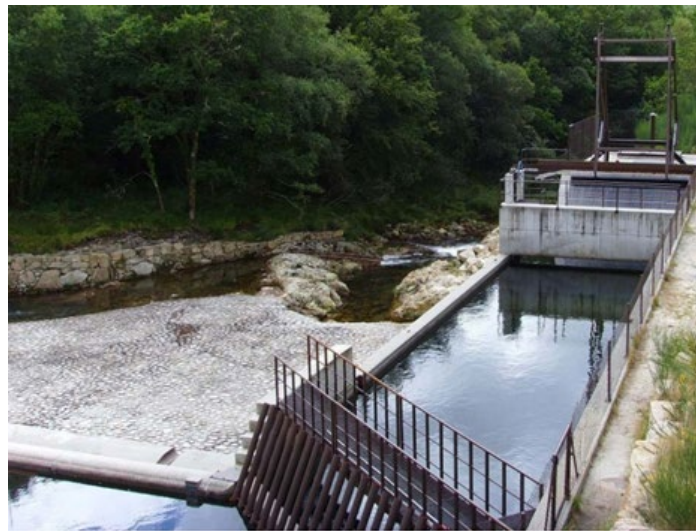
Figure 43.- Water intake with grating. Source: IDAE (2014)
