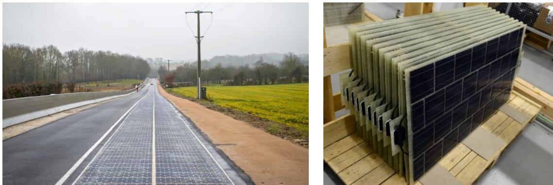
Figure 73.- Solar road in France and Wattaway panels. Source: Guardian (2016)
