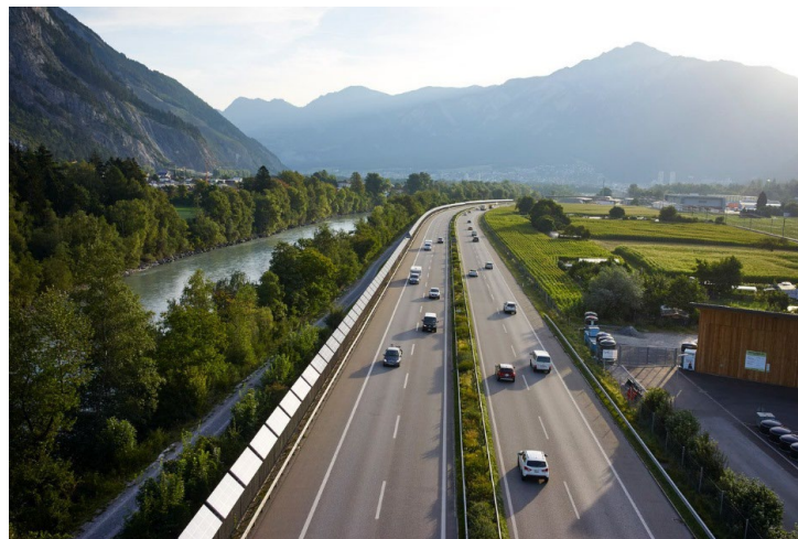
Figure 77.- PVNB in Domat/Ems (Switzerland) in 1989. Source: TNC AG
