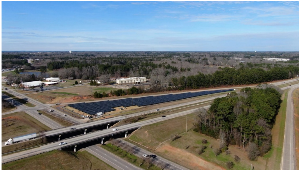
Figure 87.- Solar PV installation at the Exit 14 of the I-85 (Georgia). Source: Ray (2019)
