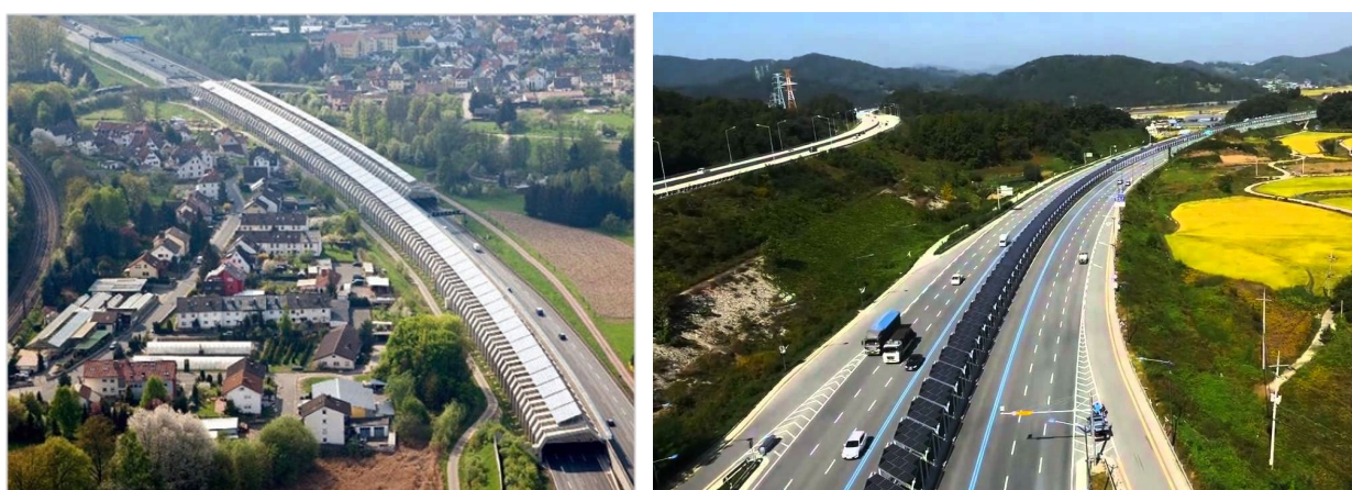
Figure 93.- Solar tunnel and bike lane in Germany and South Korea. Source: Volpe 2012
