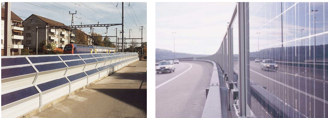
Figure 78.- PVNB in Wallisellen and Aubrugg (Switzerland). Source: Nordmann and Clavadetscher, 2004
