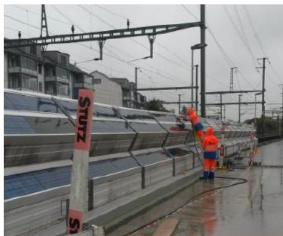
Figure 96.- Cleaning of the Wallisellen PVNB after roadworks. Source: SEAC (2015)
