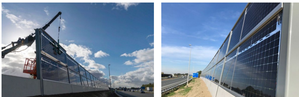
Figure 82.- PVNB in Uden. Source: Solar Highways (2021).
