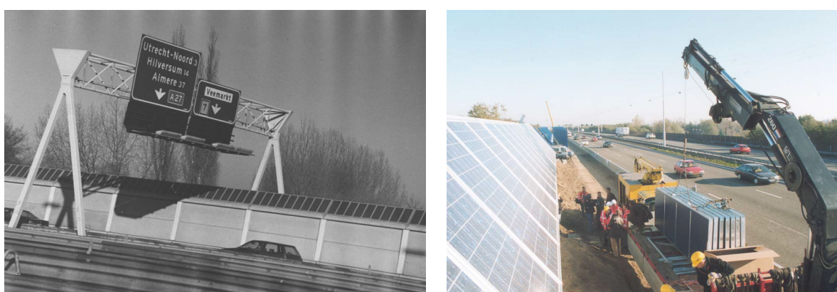
Figure 79.- PVNBs in A27 and A9 (NL). Source: Betcke et al. (2002); Nordmann and Clavadetscher (2004)
