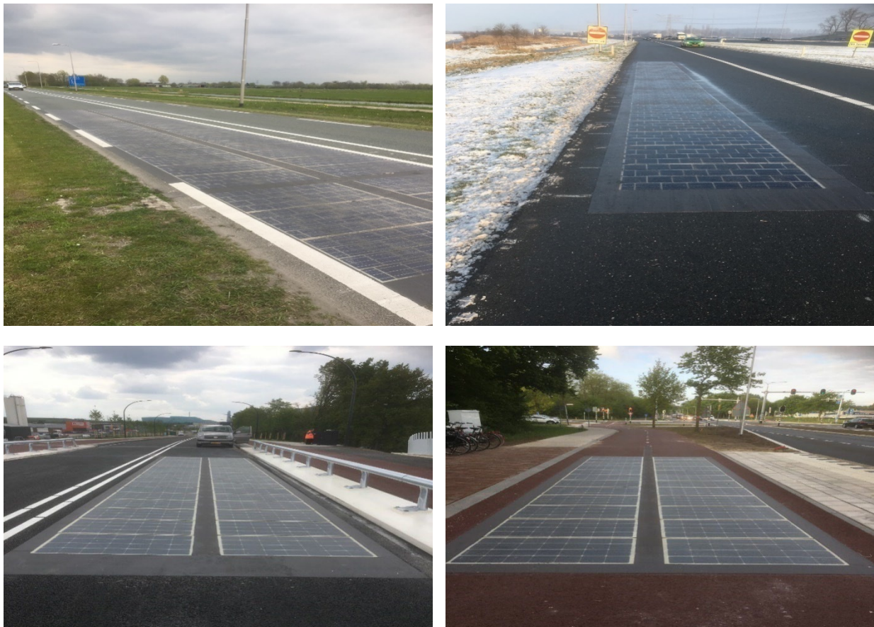
Figure 74.- N401 road, A2 motorway, Hengelo and Grave, NL (top to bottom and left to right). Source: BAM
