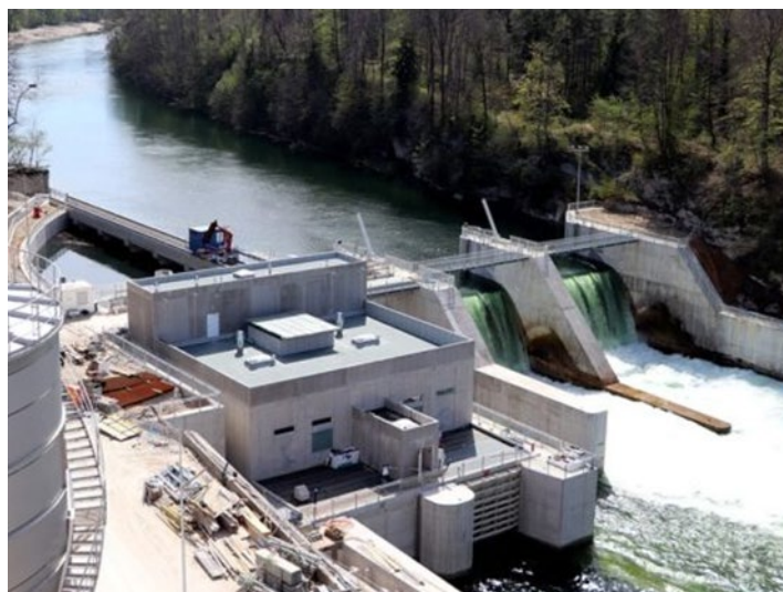
Figure 44.- Power house of a mini hydro power plant. Source: ambientum.com
