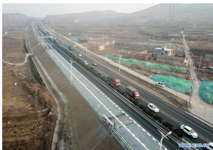
Figure 76.- Solar road in Jinan, China. Source: NSEnergy (2019)
