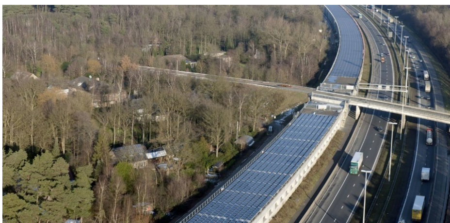
Figure 94.- High speed rail solar tunnel between in Belgium. Source: Newatlas (2011)
