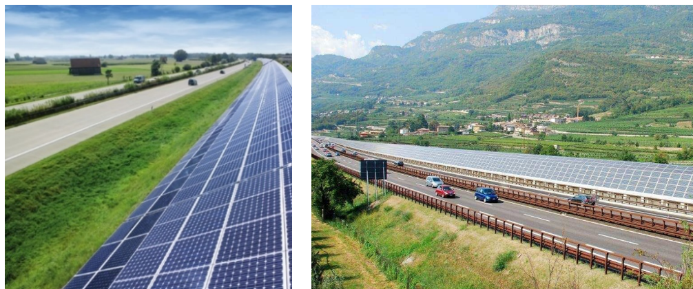
Figure 80.- PVNBs in at Fresing (Germany) and Marano (Italy). Source: Wikimedia (Isofoton)
