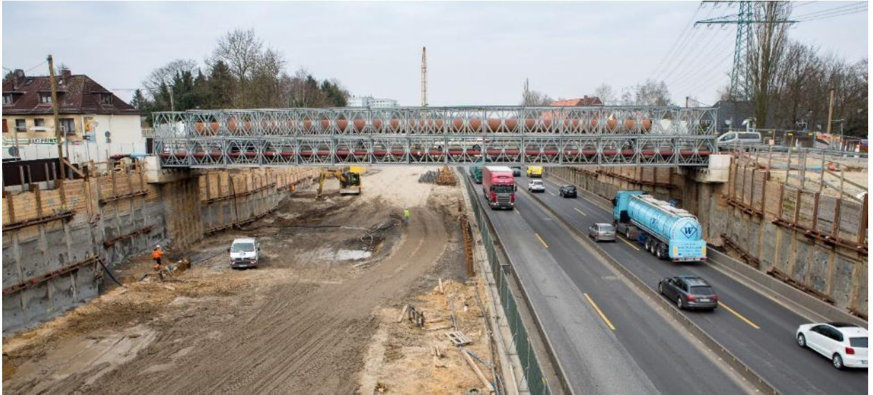
Figure 140: Situation during construction phase – traffic shifted to one side and speed limits.
