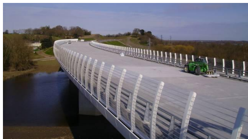
Figure 28: Sound reflecting noise barriers curved to reduce the negative effect of sound reflections
